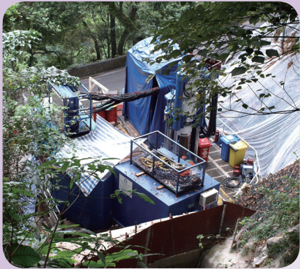
Raise Boring Machine is excavating the dropshaft at Intake M3 on May Road
