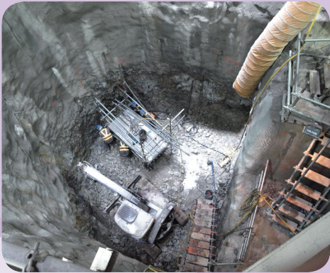
Dropshaft excavation is underway at Intake BR6 on Kennedy Road
