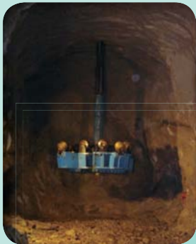
The reamer is installed to the rod.
