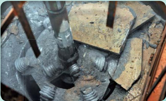
The reamer bores through the ground surface.
