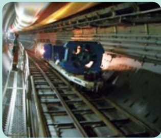
The large reamer is being transported from the main tunnel to the bottom of dropshaft.
