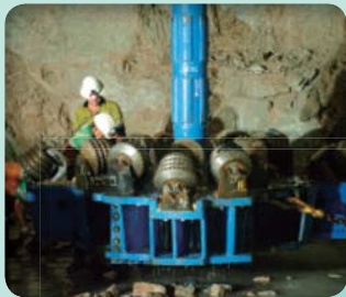
Workers install the reamer.
