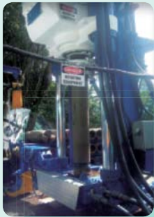
A pilot drill hole with smaller diameter is drilled down to the adit.
