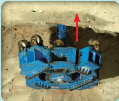
The reamer will bore upward to the ground surface and excavate the shaft along the way.
