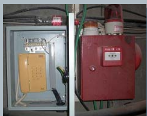
Lined telephone at each 90m along tunnel
