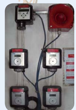
Monitoring of toxic gas such as carbon monoxide.
