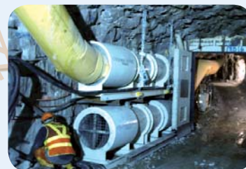
Ventilation pipes to supply fresh air to the tunnel and extract fumes from adits after blasting.
