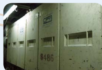
Chiller to maintain the temperature inside the tunnel.
