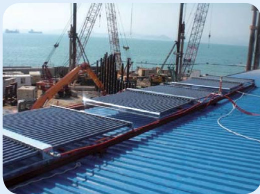
Solar panels installed at the roof of the Workshop
