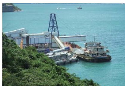
Fully enclosed conveyor system transports spoils out of the Western Portal
