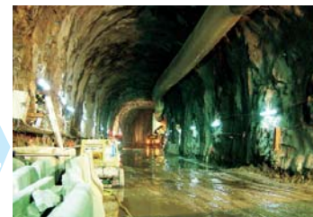
Part of the tunnel at the east is excavated by the drill and blast method
