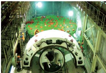
TBM assembly at Eastern Portal
