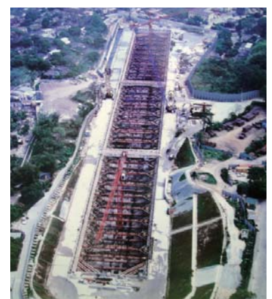
The tunnel at Kwu Tung, Sheung Shui of the MTR Lok Ma Chau Spur Line is constructed by the cut and cover method
