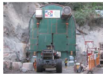
The blast protection door is closed during blasting operation
