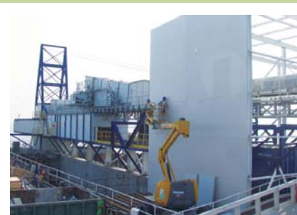
Noise barrier is erected at the Western Portal to reduce noise
