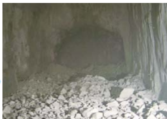
The blasting results in the rock being broken out
