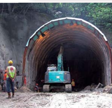
Eastern Portal - Tunnel excavation by mechanical method
