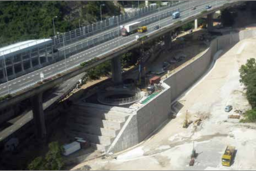
TRANSPORTATION-LEISURE-DRAINAGE THREE-FOLD LAND USE: THE STILLING BASIN BENEATH TSING SHA HIGHWAY WITH THE BASIN DECK BEING DEVELOPED INTO A PET GARDEN 防洪、康樂、運輸一地三用：位於青沙高架橋下的靜水池，上蓋建為寵物公園
