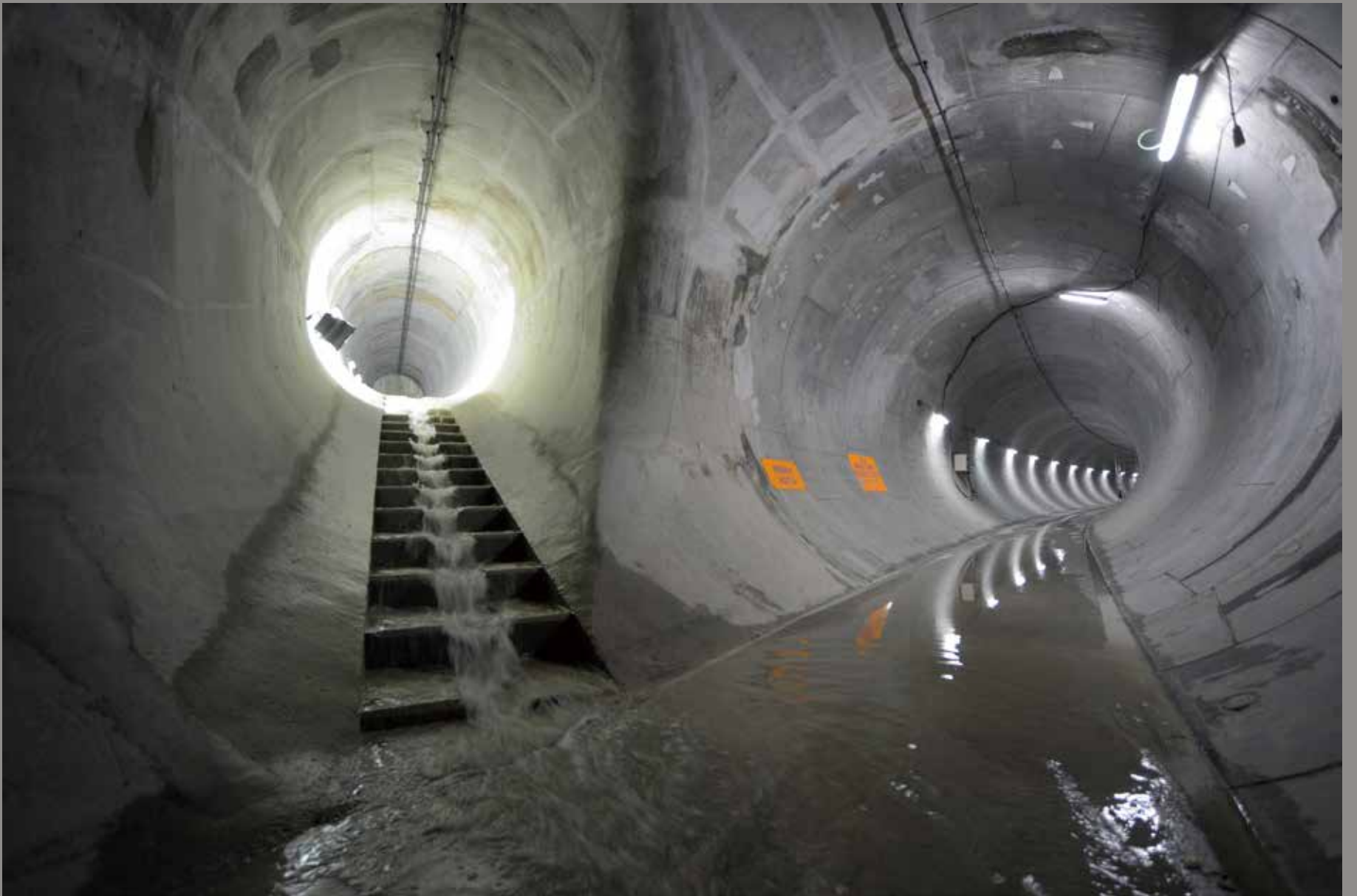
CONFLUENCE OF AN ADIT AND THE BRANCH TUNNEL 連接隧道與分支隧道交匯點
