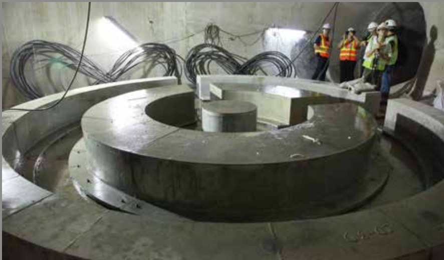
BAFFLE RING AT THE BOTTOM OF AN INTAKE SHAFT FOR TURBULENCE SUPPRESSION 進水豎井底用以減低湍流的齒環結構
