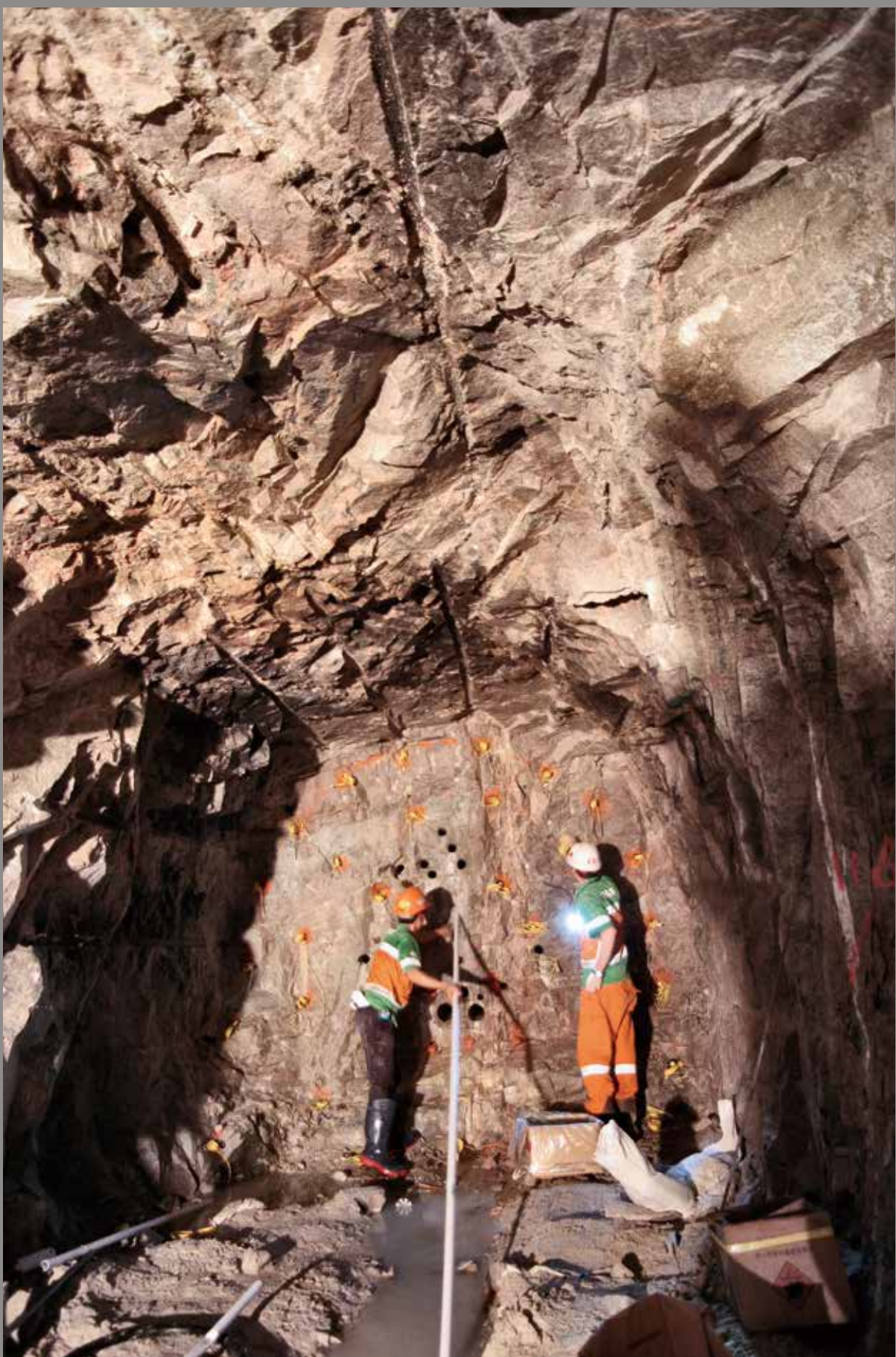
DRILLING AND BLASTING WORKS FOR ADIT EXCAVATION 以開掘方法挖掘連接隧道
