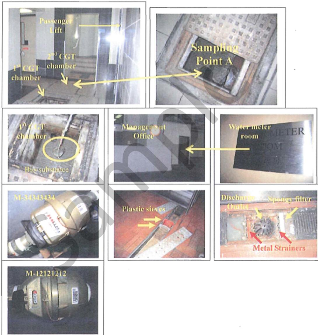
Central Grease Trap A (CGT-A) was located at the G/F car park (near the passenger lift). "Bio-substance" was placed inside the 1<sup>st</sup> chamber of the CGT. Sampling point A was at the outlet of the CGT. Water Meter Room was located at the G/F car park. The entrance of the room was beside the management office.
