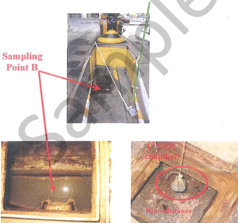
Central Grease Trap B (CGT-B) was located at the entrance of the G/F car park. "Bio-substance" was placed inside the 1<sup>st</sup> chamber of the CGT. Sampling point B was at the outlet of the CGT.
