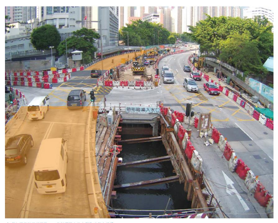
▲ 彩虹道及沙田坳道路口,位於河道上的大型臨時行車鐵橋 At the intersection of Choi Hung Road and Shatin Pass Road, a large-scale steel deck above the river course was built to enable trafficking
