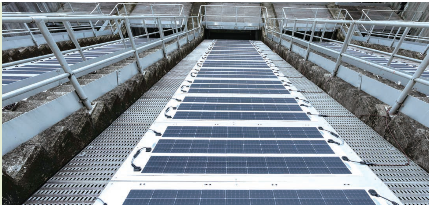
A flexible PV system installed on the covers of the screw pump channels 於泵房螺絲泵槽上蓋安裝的柔韌式太陽能板
