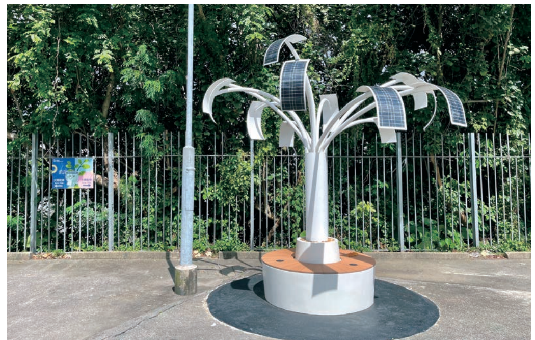
A solar tree installed within the pumping station to produce renewable power from solar energy 在泵房範圍內安裝一棵太陽能樹，利用太陽能產生可再生能源
