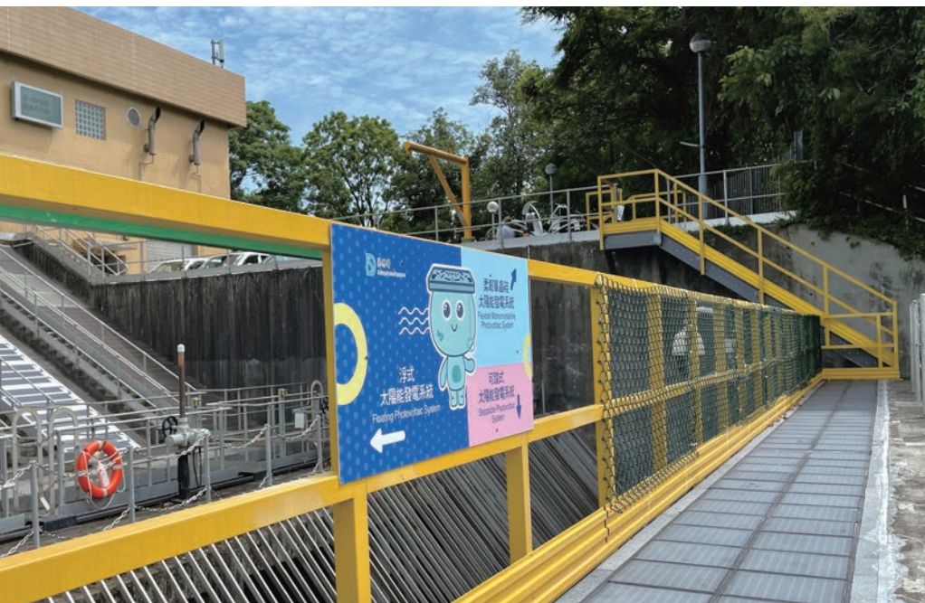
A steppable PV system installed on maintenance platform 於泵房內維修平台安裝的可踏式太陽能板
