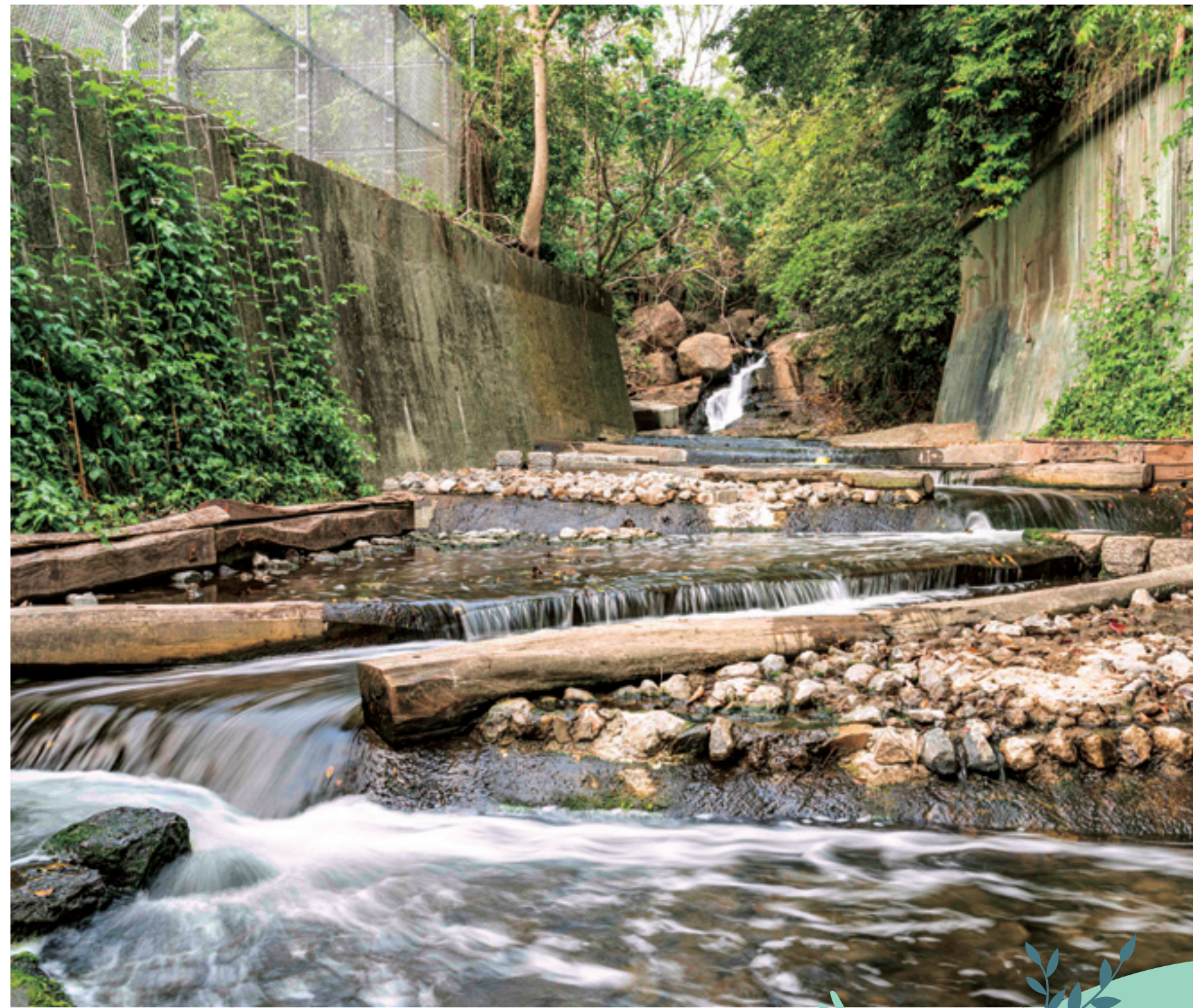
▲ 15 shoals and 15 fish ladders were built, intended as resting area for fishes and other aquatic species. 我們建造了約15個淺灘及15條魚梯，提供空間讓魚類和其他水生動物逗留。
