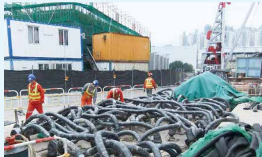
Insulated delivery and return pipes 輸送和回流的絕緣喉管
