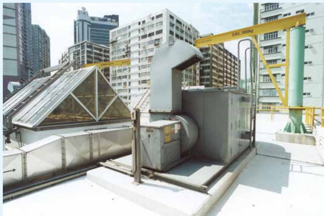
Air extraction system complete with modular activated carbon type deodourisation units on the roof top of Chai Wan PTW
