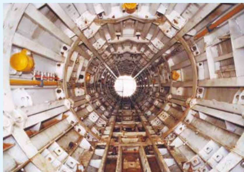
Tunnel formwork in Tunnel F from Tsing Yi to Stonecutters Island 由青衣至昂船洲隧道F的隧道模板
