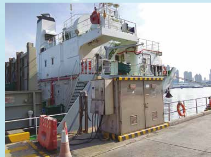
Connected to on-shore power supply when berthed 泊岸時連接岸上的電源
