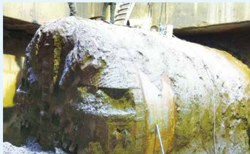
Breakthrough by tunnel boring machine "Victoria" at inlet chamber 隧道鑽挖機「維多利亞」貫通進水室
