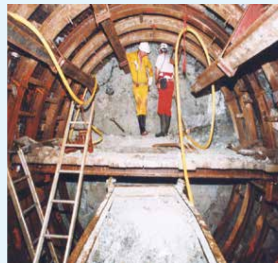
Manual excavation through Lead Mine Pass Fault in Tunnel F from Chainage 744 to Chainage 760 隧道F經過鉛礦坳斷層由744至760段的人手挖掘情況
