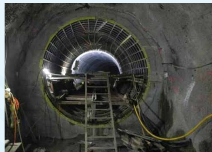
Concrete lining completed 混凝土襯砌完成
