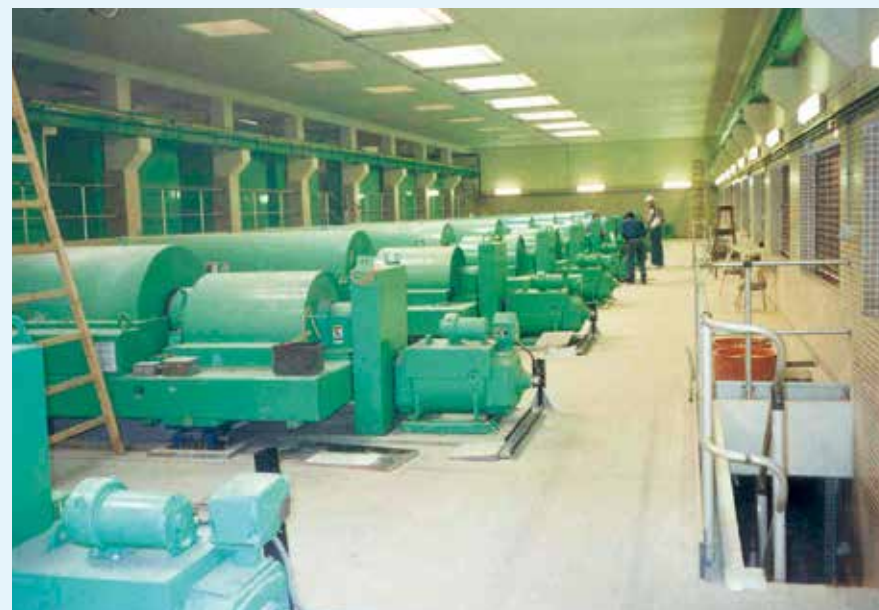
Centrifuges in sludge dewatering facility 污泥脱水设施内的离心机
