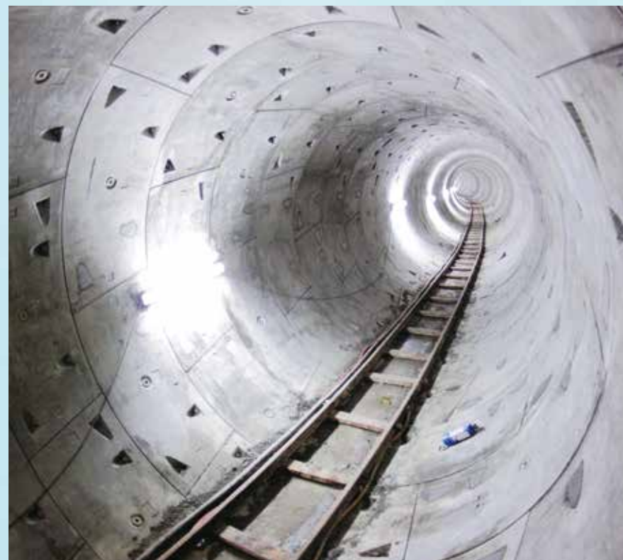
Interior structure of interconnection tunnel 連接隧道內部結構
