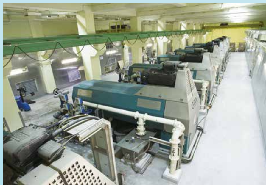
Centrifuges inside the sludge dewatering building 污泥脱水大樓內的離心機
