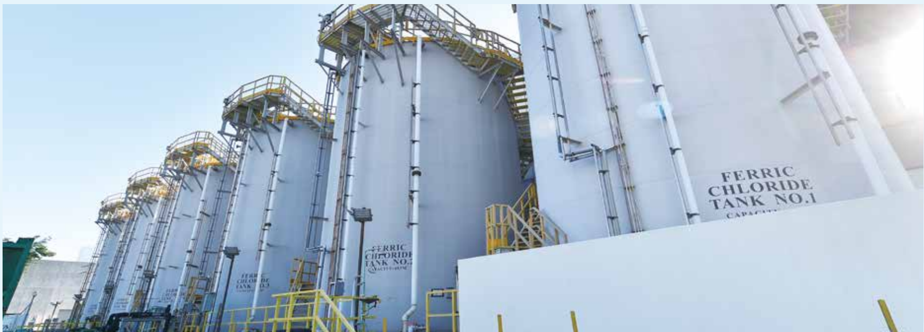
Ferric chloride storage tanks 三氯化鐵儲存缸
