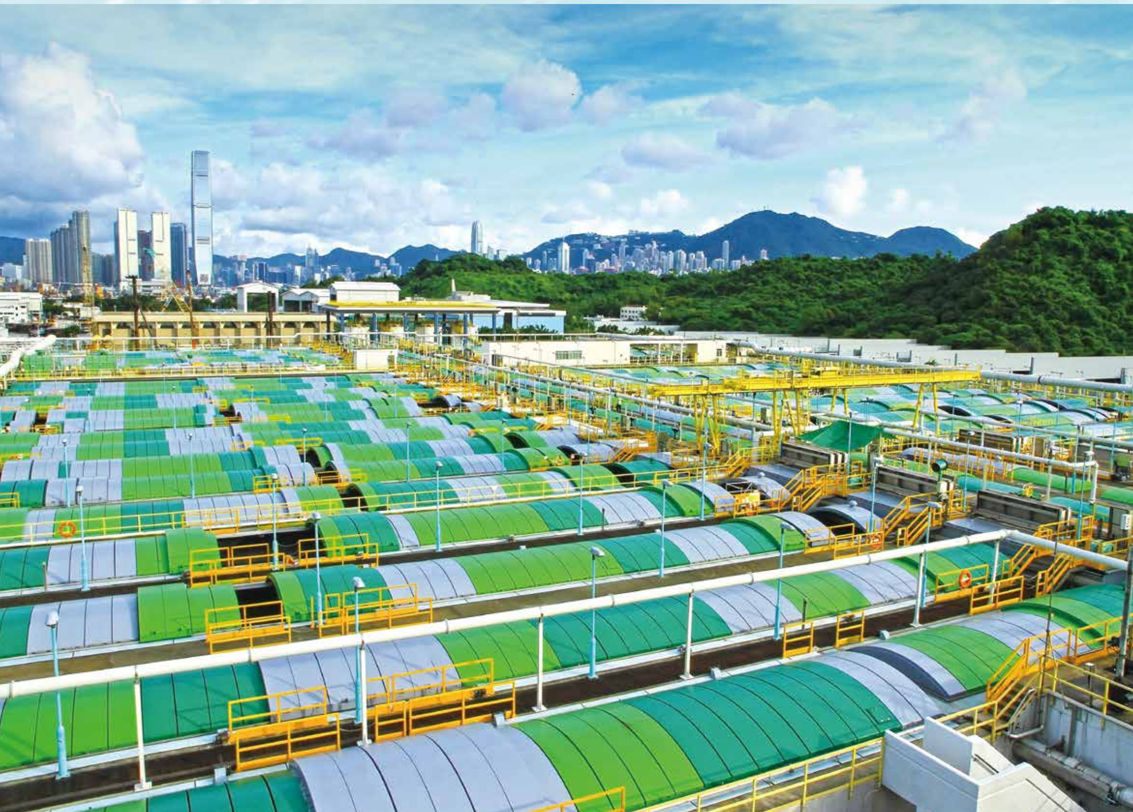
Double-decked sedimentation tanks with fibre-glass covers 雙層沉澱池以玻璃纖維罩覆蓋
