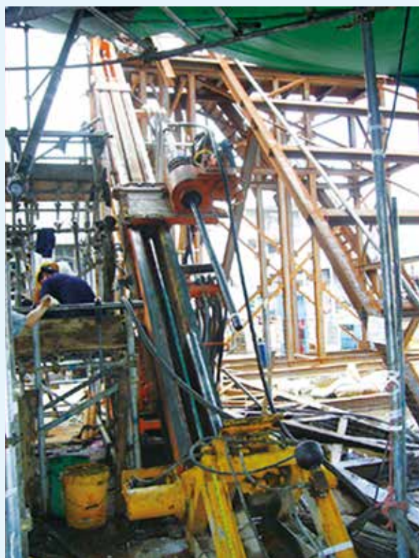
Setup for directional coring 定向取芯設置
