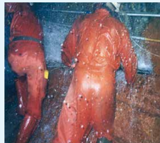
Serious water inflow in Tunnel F from Kwai Chung to Tsing Yi 由葵涌至青衣的隧道F地下水湧入情況嚴重
