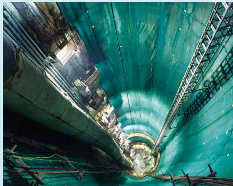
Shaft connecting deep sewage tunnel under construction 連接深層污水隧道的豎井在建造中
