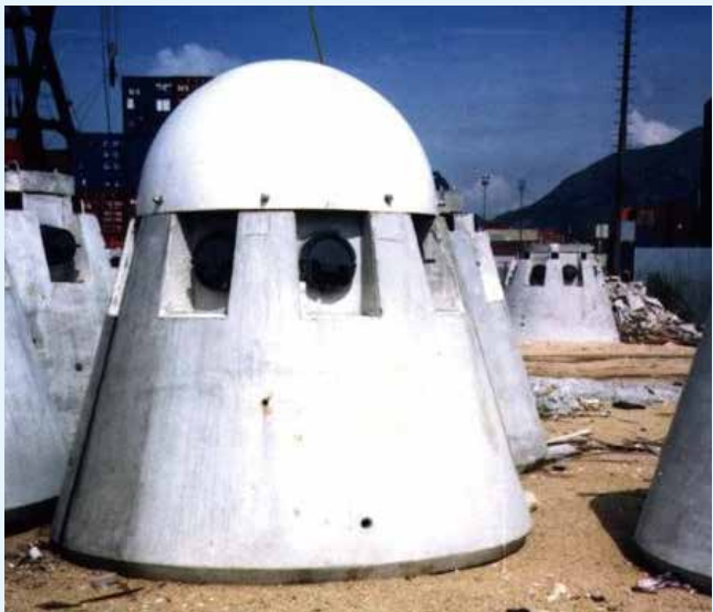
Diffuser head with protective dome 擴散器頂部加裝了保護圓罩
