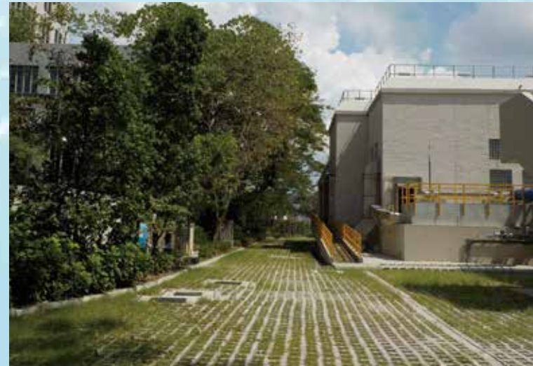
Permeable pavement with grasscrete panels at North Point PTW 北角基本污水處理廠的透水性鋪面及混凝土草格
