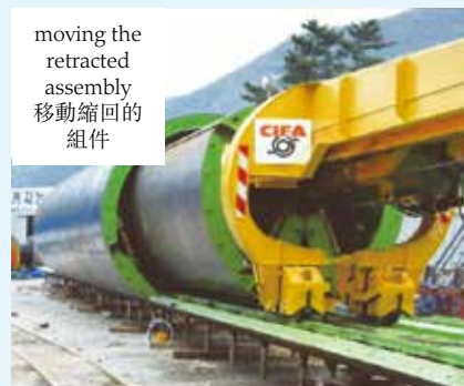
Telescopic lining formwork 伸縮式模板裝置
