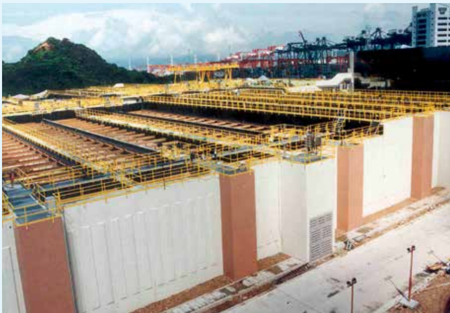
Double-decked sedimentation tanks 雙層沉澱池
