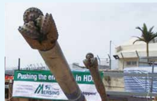
Completion of pilot hole drilling 完成鑽挖導孔
