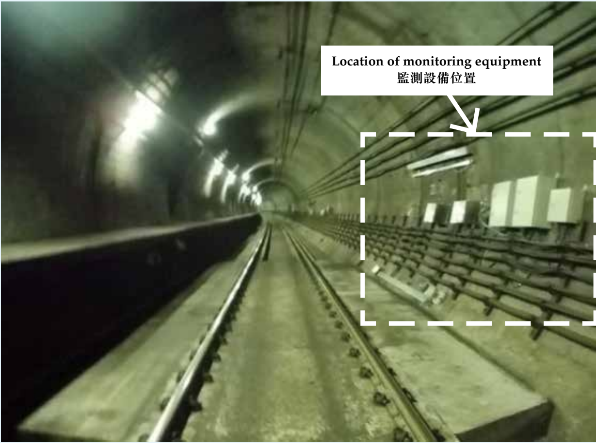
MTR tunnels monitoring equipment 港鐵隧道監測設備
