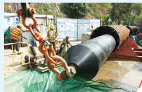
Completion of pipe pulling 完成拉喉工序
