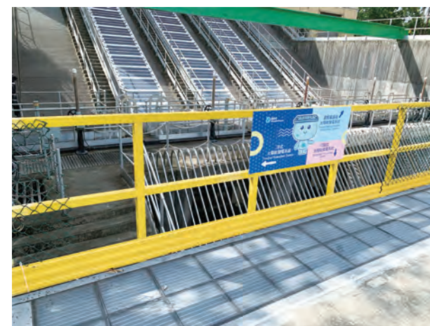
▲ 安裝於新田雨水泵房內維修平台的可踏式太陽能發電系統 Steppable photovoltaic systems (PV) was laid on top of the maintenance platform at San Tin Stormwater Pumping Station
