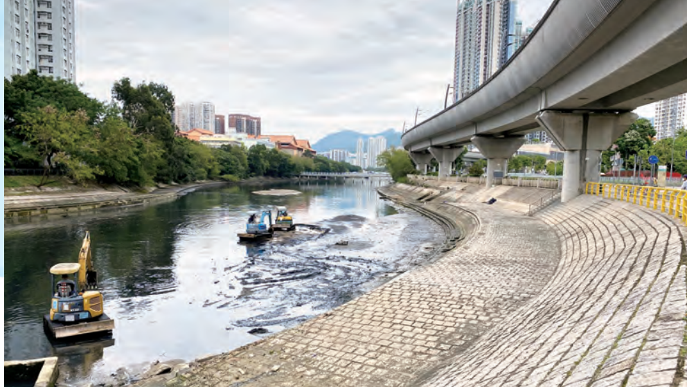
◀ 渠務署於城門河近文禮閣進行清淤工作 Drainage desilting works by the DSD at Shing Mun River near Man Lai Court
