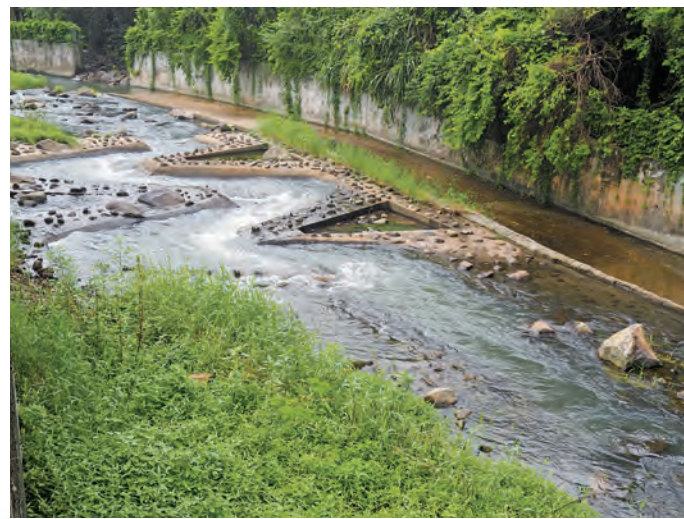
▲ 林村河上游三條「之」字型設計的魚梯，上設凹位，供魚類棲息 Three zig-zag fish ladders in Upper Lam Tsuen River designed with still water troughs to provide refuge for fish
