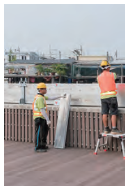
▲ 於大澳沿岸安裝可拆卸式擋水板 Demountable flood barriers installed along the coast of Tai O
