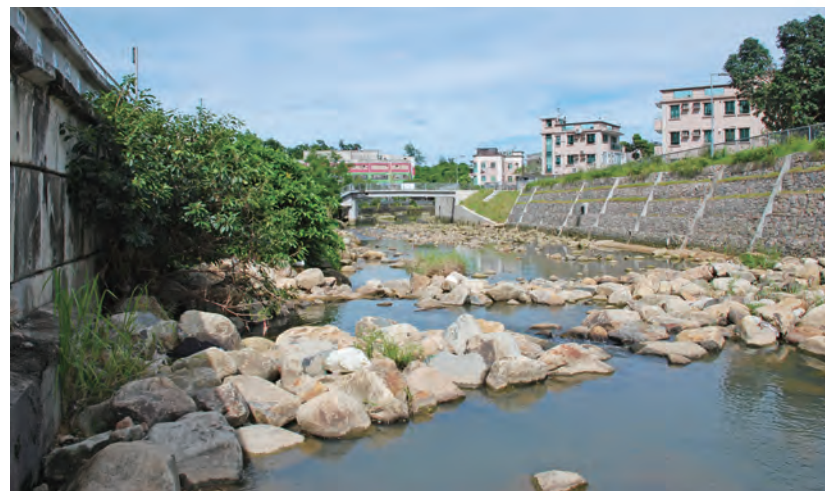
▼ 蠔涌河河道改善工程於2017年完成，圖為蠔涌河由不規則的石塊和卵石形成的魚梯 Ho Chung River Improvement Works was completed in 2017. Image displays fish ladders laid by passage of boulders and cobbles in Ho Chung River
