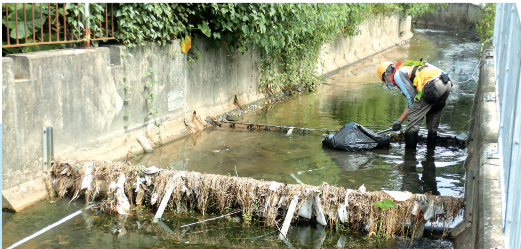
▼ 前線員工於西貢井欄樹進行清理渠道工作 Frontline staff cleaned and desilted drains at Sai Kung Tseng Lan Shue
