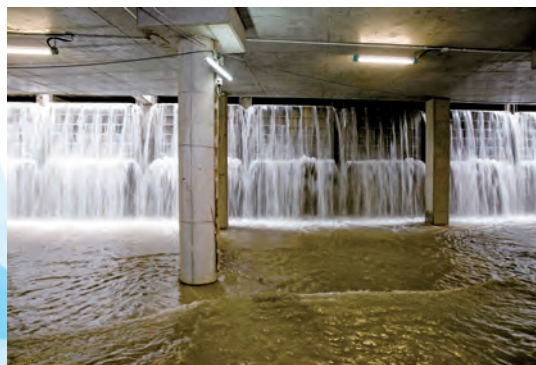
▲ 跑馬地地下蓄洪計劃分兩期進行，分別於2015年及2017年投入運作。圖為跑馬地地下蓄洪池智能水閘的操作示範 Happy Valley Underground Stormwater Storage Scheme (HVUSSS), implemented in two phases, was commissioned in 2015 and 2017 respectively. Image displays the demonstration of Movable Weir operation at HVUSSS
