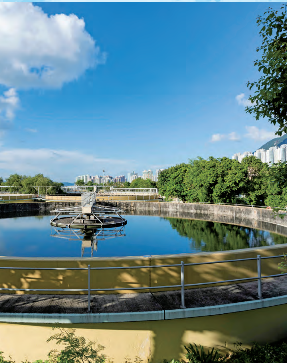
▲ 沙田污水處理廠的圓形最後沉澱池 Circular shaped final sedimentation tank at Sha Tin Sewage Treatment Works
