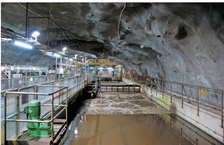
▼ 赤柱污水處理廠建於三個岩洞內，每個約120米長、15米寬和17米高，並由 超過450米的通道、通風隧道及豎井連接，是東南亞首間建於岩洞內的污水 處理廠 Stanley Sewage Treatment Works is housed inside three caverns, each about 120 metres long, 15 metres wide and 17 metres high together with over 450 metres of access roads, ventilation tunnels and shafts. It is the first sewage treatment works built in caverns in Southeast Asia
