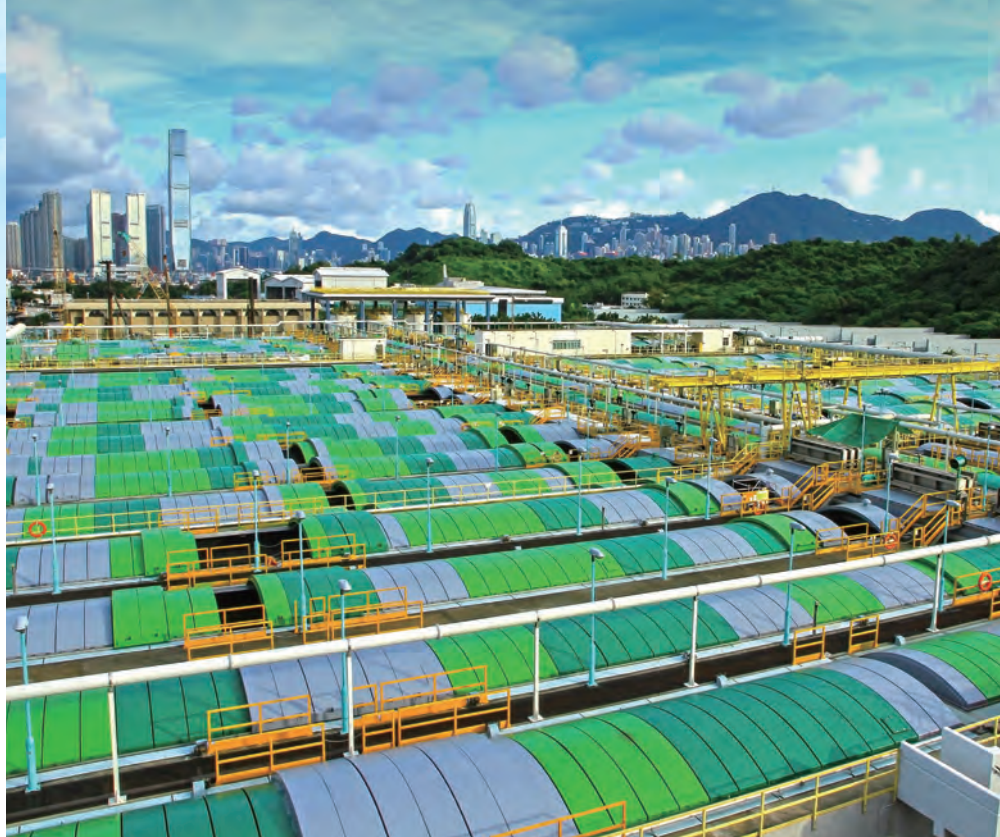
◀ 昂船洲污水處理廠化學強化一級處理沉澱池 Sedimentation tanks for chemically enhanced primary treatment at SCISTW
