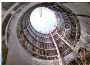
▲ 啟德轉運計劃於2004年落成啟用，計劃包括建造一條1.43公里長的雨水隧道，圖為建造中的豎井 Kai Tak Transfer Scheme, which commenced in 2004, comprises the construction of a 1.43-kilometre-long drainage tunnel. The image displays a "drop shaft" under construction
