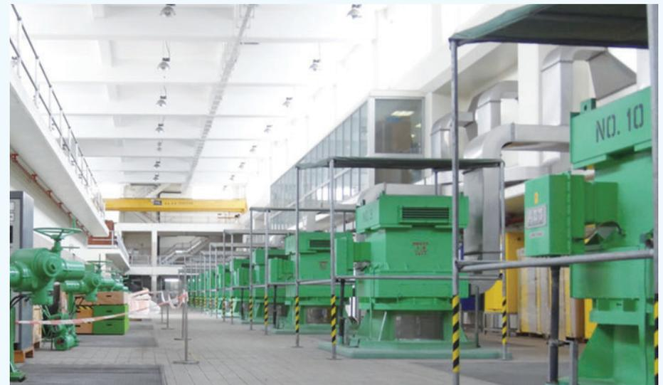
3.3 kilovolts high-voltage centrifugal sewage pump in the Cheung Sha Wan Sewage Pumping Station
