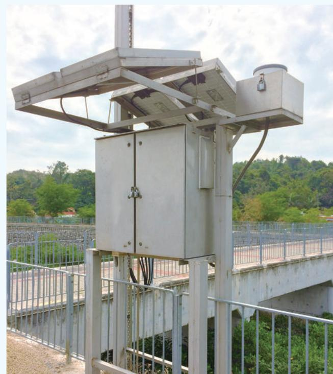
A remote-controlled gauging station equipped with solar panel, rain gauge and water level sensor for real-time monitoring.
