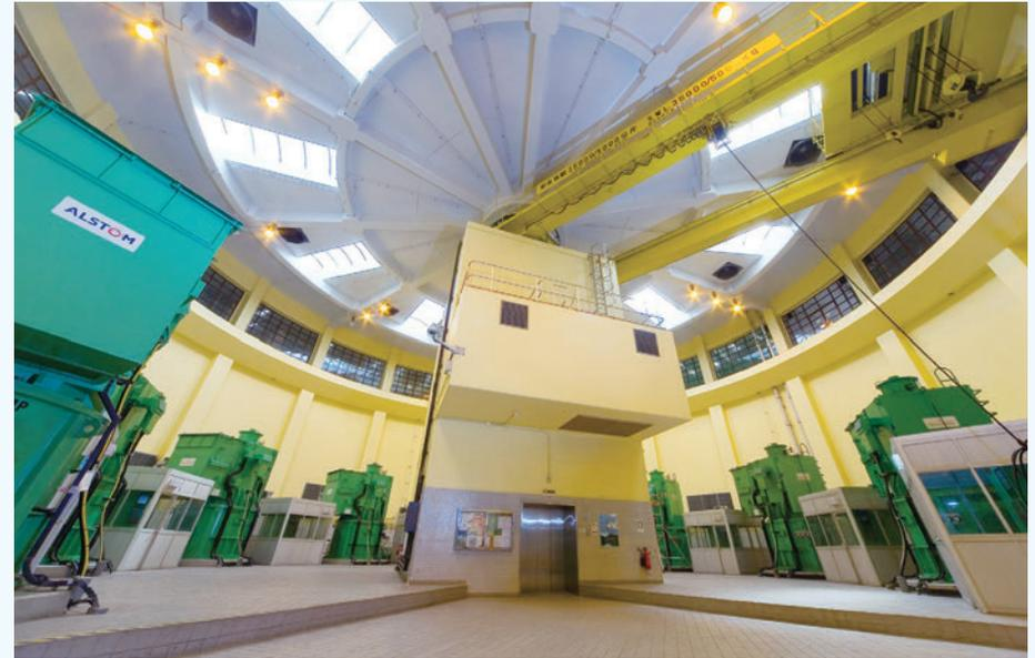
Eight sewage pump motors installed in the Main Pumping Station No. 1 at the Stonecutters Island Sewage Treatment Works under the Harbour Area Treatment Scheme
