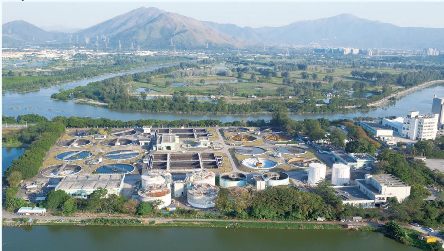
The DSD has planned to upgrade the Yuen Long Sewage Treatment Works to effluent polishing plant with tertiary treatment
