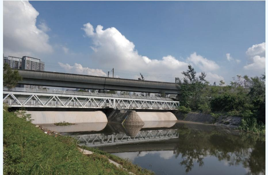
Inflatable dam at San Tin Eastern Main Drainage Channel near its confluence with Shenzhen River, the highest inflatable dam in Hong Kong with a 5 metres full height.
