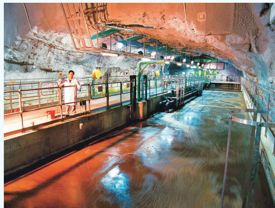
The wastewater collection, treatment and disposal systems under the Hong Kong Island South Sewerage Master Plan include a secondary treatment works at Stanley built inside cavern.
