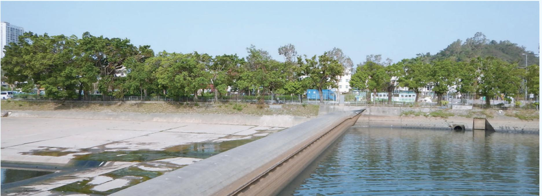
Inflatable dam in Yuen Long Main Nullah near Tung Tau Wai was constructed in 1992 to prevent polluted tidal water from backflowing into the Yuen Long town centre
