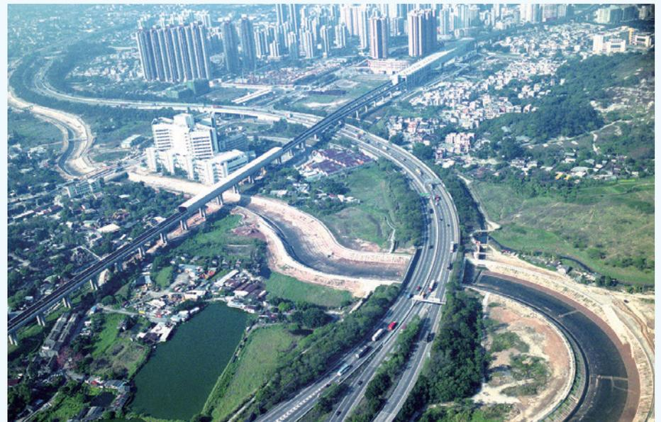
Yuen Long Bypass Floodway diverted part of the runoff from Yuen Long town centre to Kam Tin River east of Yuen Long to reduce the risk of flooding in the Yuen Long Town
