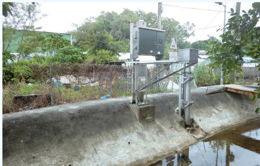
The DSD has installed flood alarm systems to alert the local villagers at flood-prone areas before drainage improvement works are completed
