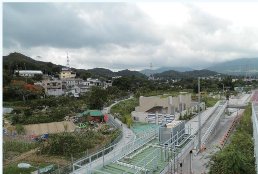
Sewage pumping stations are constructed in some village sewerage projects to convey wastewater
