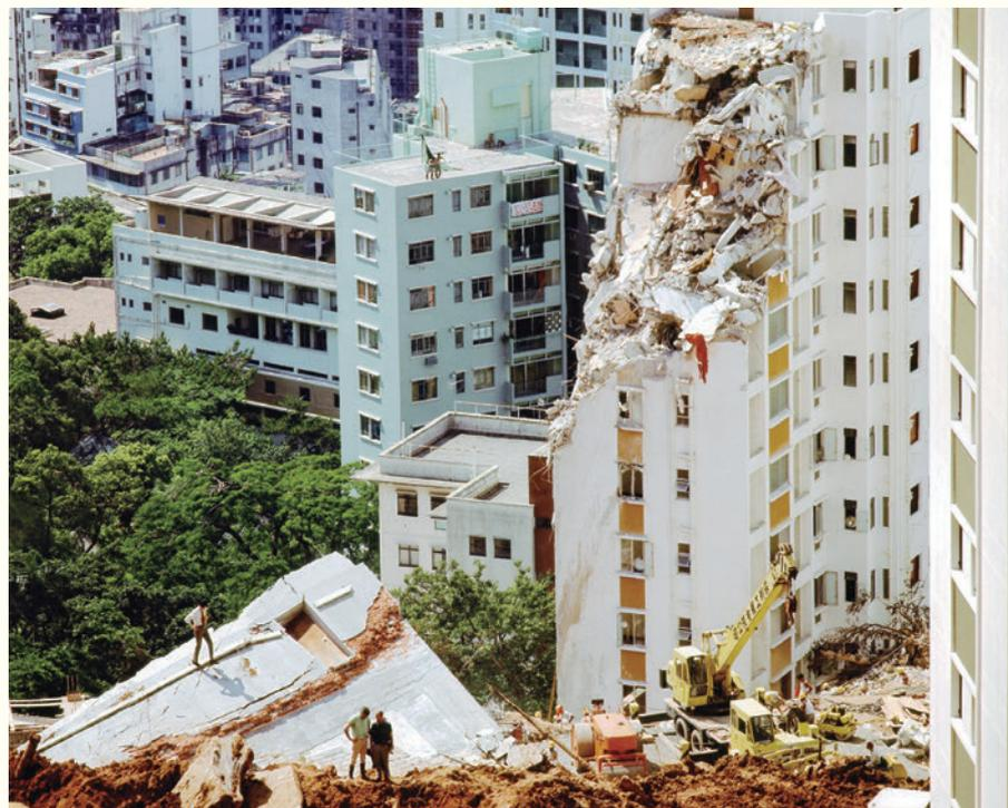
Remains of two buildings at Kotewall Road, following the devastating landslide that occurred on 18th June 1972. 40 000 cubic meters of rocky debris unearthed in this slip.
