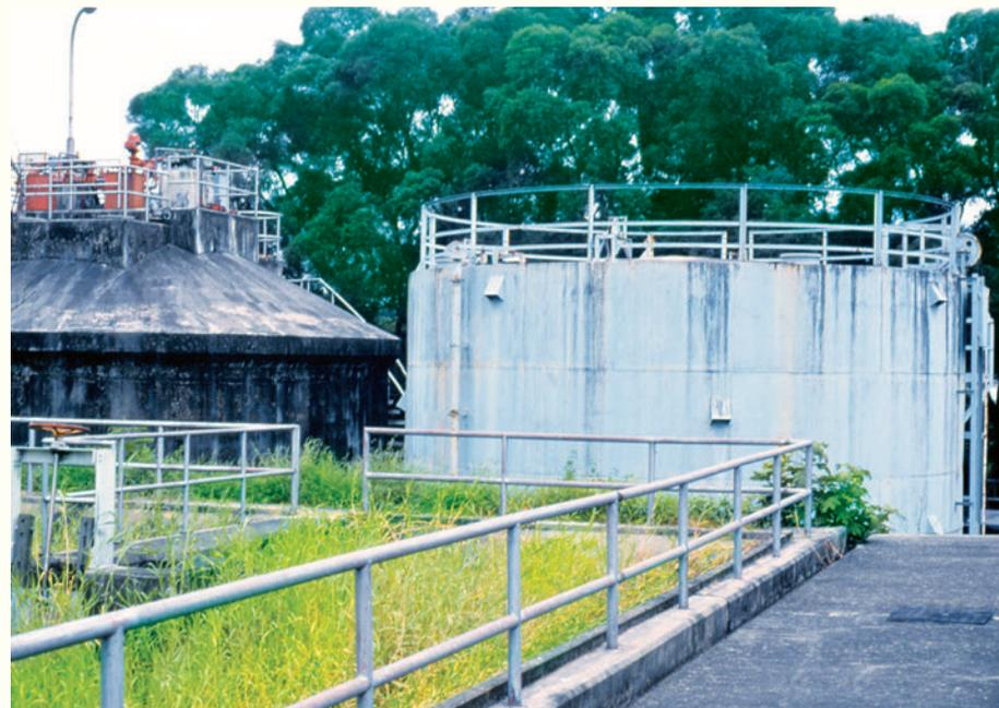
Anaerobic Sludge Digester of the Shek Wu Hui Pilot Secondary Sewage Treatment Plant
