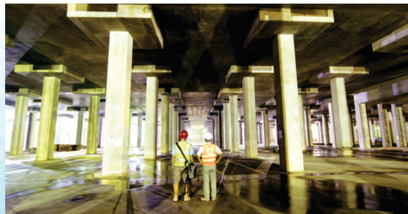
Inside view of Tai Hang Tung Underground Stormwater Storage Tank
