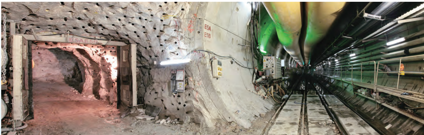
The excavation for the main tunnel and blasting operations for the connection adit were performed simultaneously
