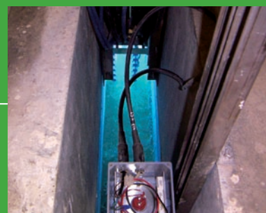
紫外光消毒槽 UV Disinfection Channel
