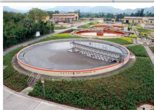
Sewage enters the primary sedimentation tank after preliminary treatment.
