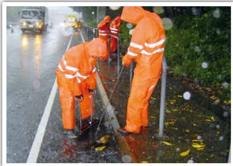
Drainage Services Department workers are clearing the blocked drains.
