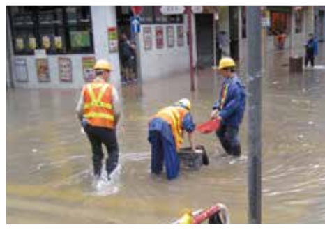
Drainage Services Department workers are clearing a blocked drain
