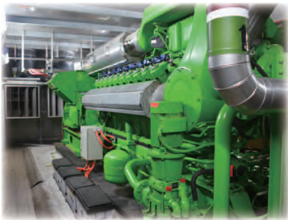
Combined heat and power generator at STSTW
