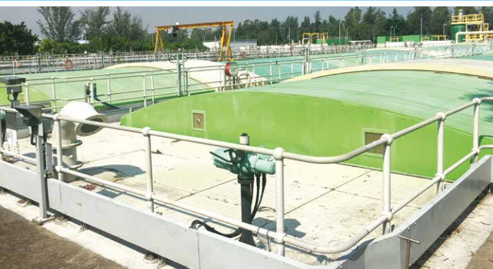
小蠔灣污水處理廠初級沉澱池的密封玻璃纖維強化塑膠蓋 Fiberglass reinforced plastic covers for primary sedimentation tanks at Siu Ho Wan Sewage Treatment Works
