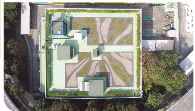
紅磡灣污水泵房 Hung Hom Bay Sewage Pumping Station
