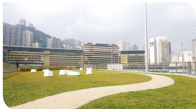
跑馬地地下蓄洪計劃 Happy Valley Underground Stormwater Storage Scheme
