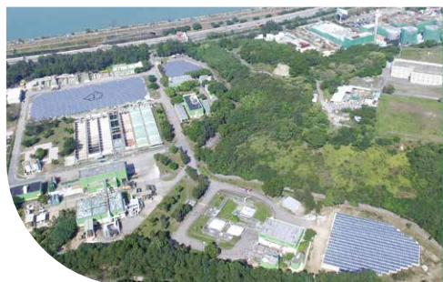
小蠔灣污水處理廠鳥瞰圖 Aerial Photo of Siu Ho Wan Sewage Treatment Works
