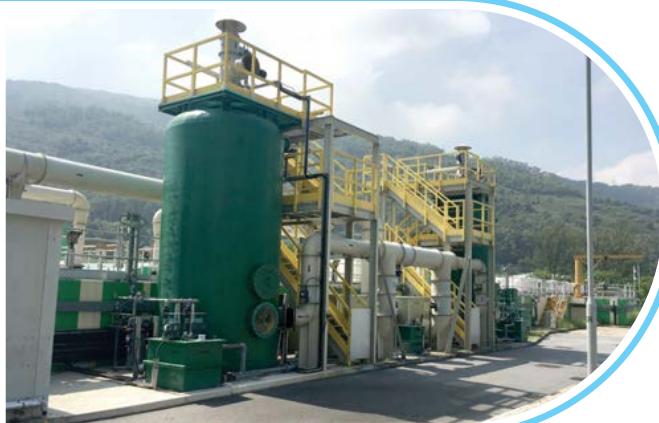
生物滴濾塔 Biotrickling filters
