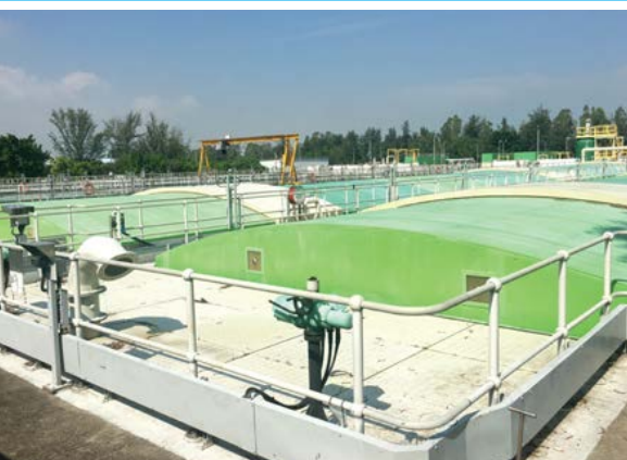
初級沉澱池的密封玻璃纖維強化塑膠蓋 Fiberglass reinforced plastic covers for primary sedimentation tanks
