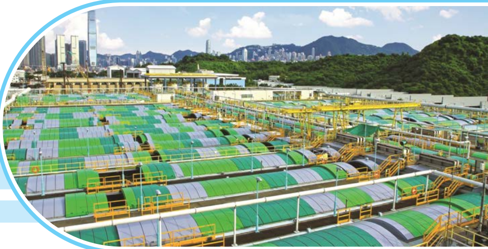
昂船洲污水處理廠一已覆蓋的沉澱池 SCISTW - sedimentation tanks with covers
