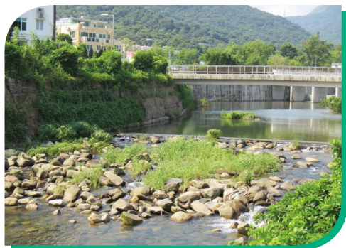
《河道設計的環境和生態考慮指引》中列舉的例子：蠔涌河（左）及白銀鄉河（右）的魚梯 Illustrative cases in the Practice Note: fish ladders in Ho Chung River (left) and Pak Ngan Heung River (right)
