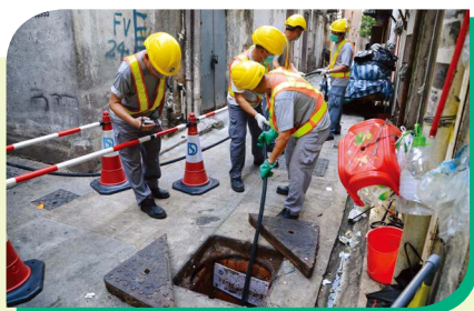
直屬員工隊以高壓噴水法清理渠管 Direct Labour Force clearing drains with water jetting
