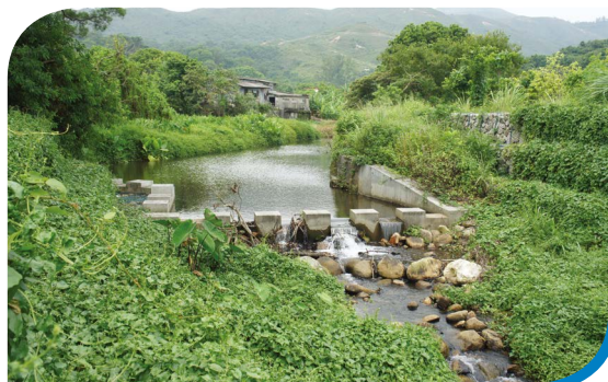
《河道設計的環境和生態考慮指引》中列舉的例子：蠔涌河（左）及白銀鄉河（右）的魚梯 Illustrative cases in the Practice Note: fish ladders in Ho Chung River (left) and Pak Ngan Heung River (right)
