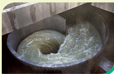
灣仔東基本污水處理廠的污水轉流到旋渦型豎井 Sewage flow diverted to the vortex dropshaft at Wan Chai East PTW
