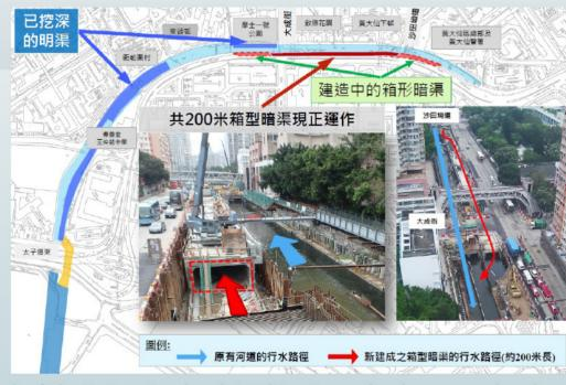
at the section between the south of Shatin Pass Road and Tai Shing Street, has been completed and a major portion of river bed in the midstream section have been deepened. The drainage capacity of the Kai Tak River has been increased before the onset of this wet season.
