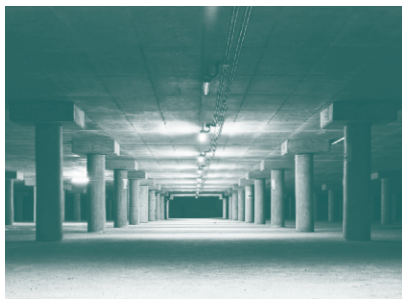
蓄洪：跑馬地地下蓄洪池 Flood Storage: Happy Valley Underground Stormwater Storage Tank
