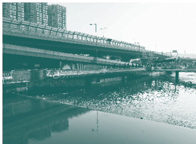
疏浚：翠屏河 Drainage Improvement: Tsui Ping River
