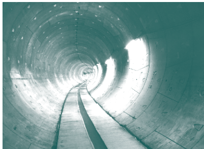
截流：雨水排放隧道 Interception: Drainage Tunnel
