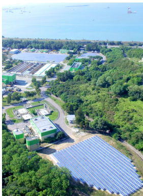
Solar Farm at Siu Ho Wan Sewage Treatment Works
