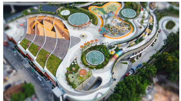
The landscaped deck built atop the roof of the Kwun Tong Sewage Pumping Station
