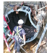
Rehabilitation Works Using Spirally-wound Liner Method
