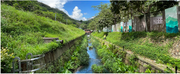
Jordan Valley Channel after revitalisation
