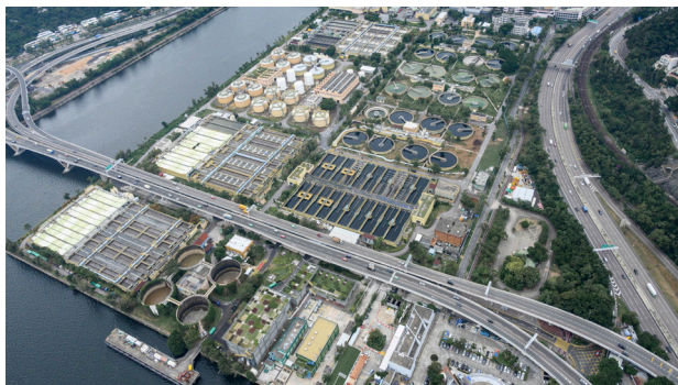
Sha Tin Sewage Treatment Works
