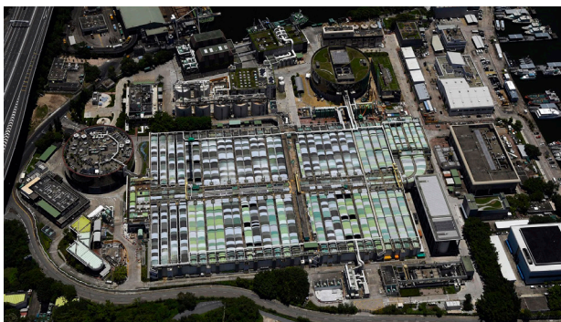
Stonecutters Island Sewage Treatment Works
