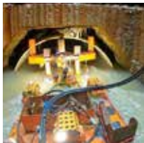
Deploying Robotic Machine for Lining Installation Works in the Existing Box Culvert with Live Sewage Flow
