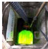
Rehabilitation Works Using UV-CIPP Lining Method
