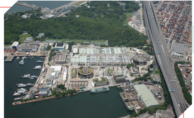
Stonecutters Island Sewage Treatment Works
