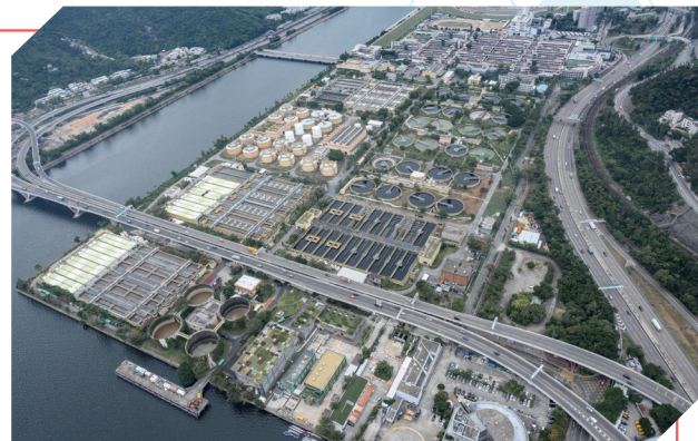
Sha Tin Sewage Treatment Works
