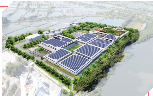
Illustration of the Completed Yuen Long Effluent Polishing Plant
