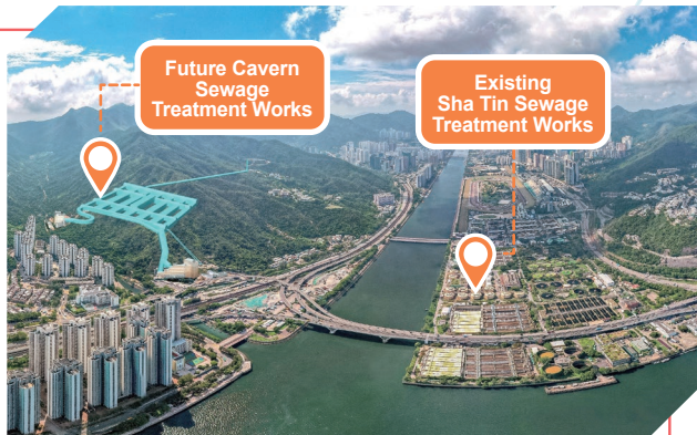
Sha Tin Sewage Treatment Works and Future Cavern Sewage Treatment Works
