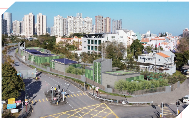
Illustration of Sha Tau Kok Underground Stormwater Storage Tank and Stormwater Pumping Station
