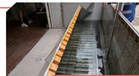
Hydrodynamic Auto Flip-up Barrier
