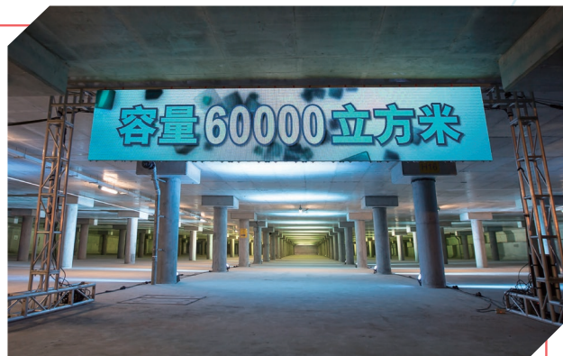
Happy Valley Underground Stormwater Storage Scheme
