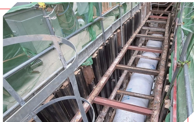
Drainage Improvement Works at Yee Fung Street, Chai Wan
