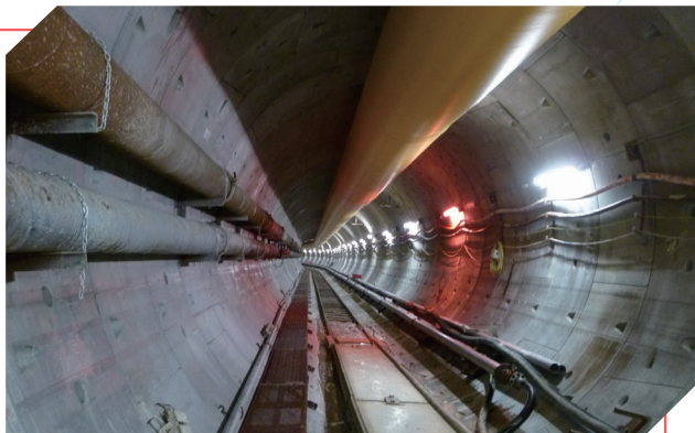
Lai Chi Kok Drainage Tunnel
