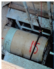
Rehabilitation of Pipe using Semi-Automated Pipe Jacking Method
