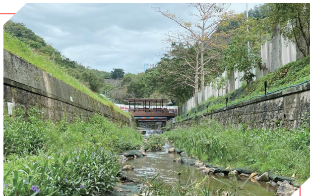
Jordan Valley Channel after revitalisation
