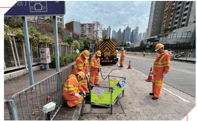
Clearing the blockage of the stormwater drains
