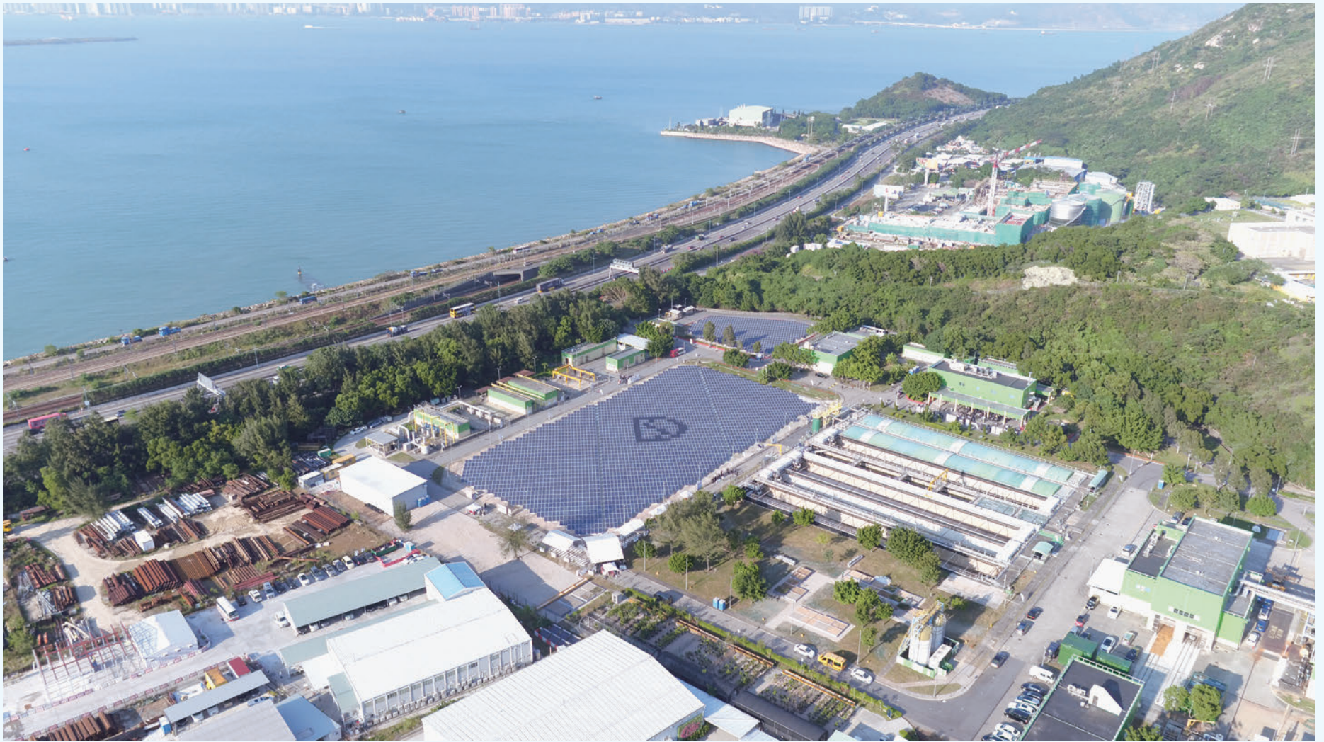
The Siu Ho Wan Sewage Treatment Works located alongside the North Lantau Highway
