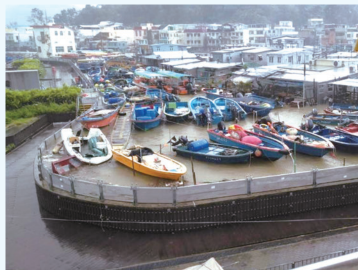
The low-lying village houses in Tai O effectively protected by demountable flood barriers installed along the river wall at times of high storm surges
