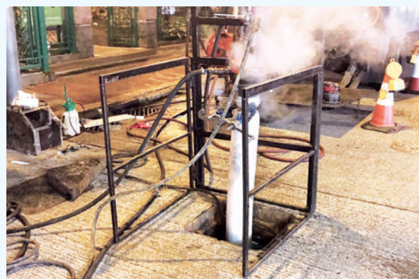
A lining is being steam-cured
