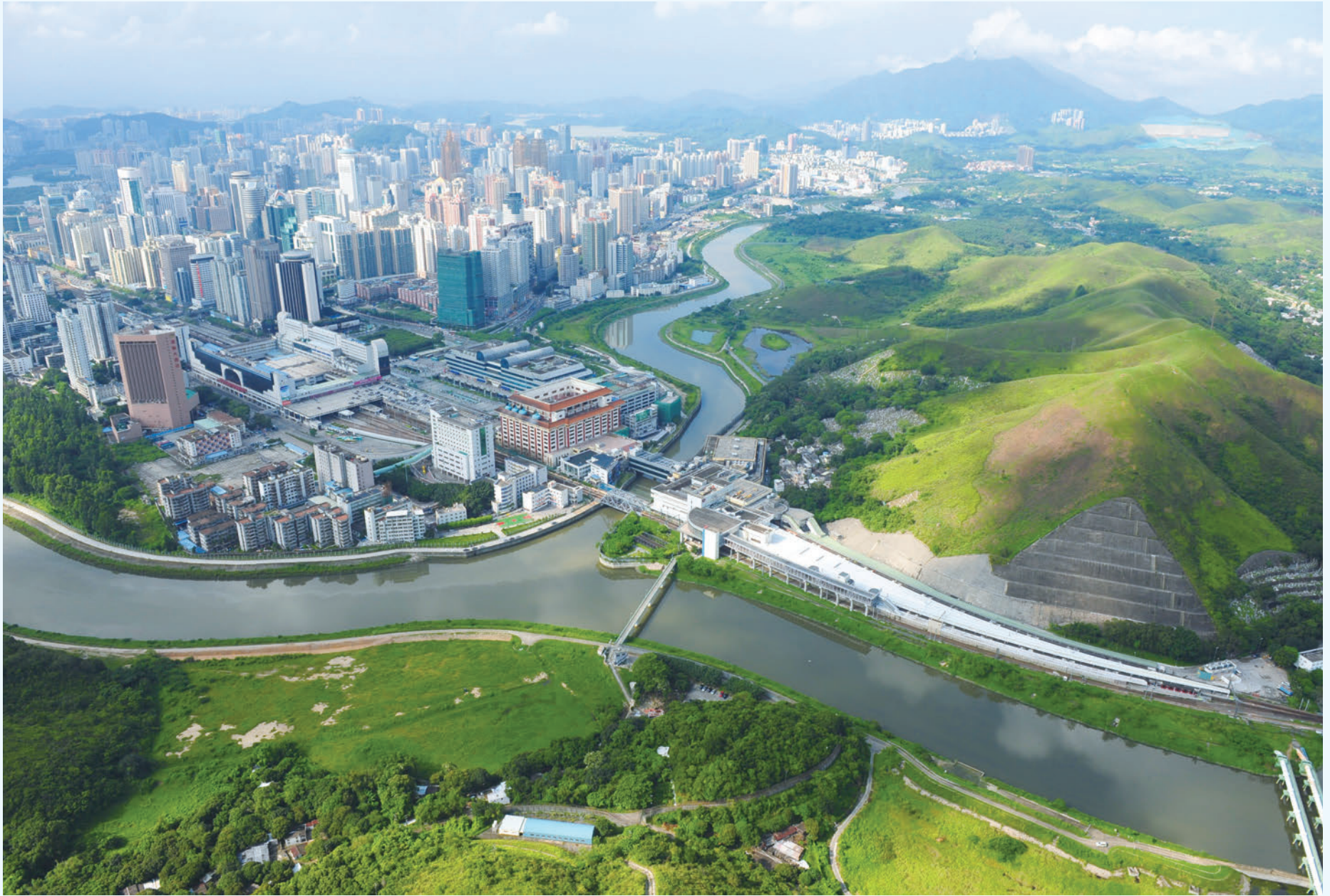
A glimpse of Shenzhen River at Lo Wu Control Point after Stage 3 works. The span of the new Lo Wu railway bridge was extended from 32 metres to 40 metres.
