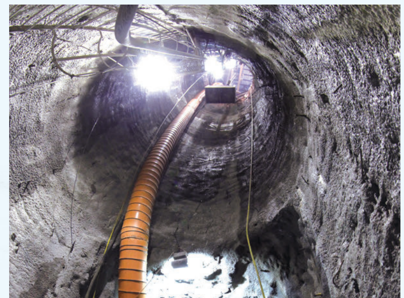
Construction of the intake shaft for the drainage tunnel
