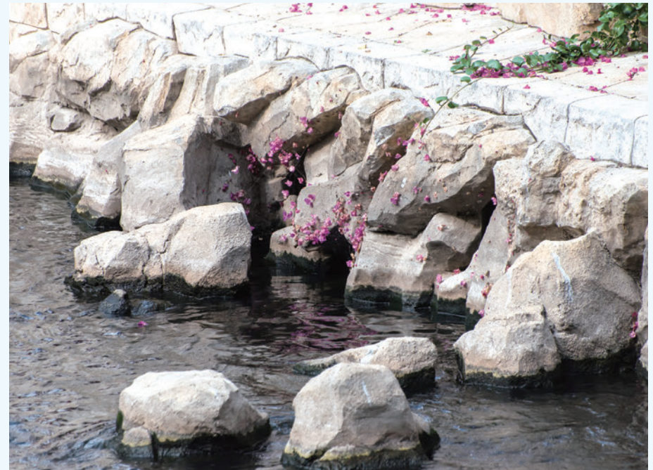
Fish shelters and deflector stones at the Kai Tak River provide habitats for marine creatures
