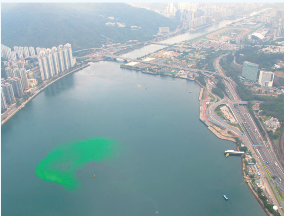
Dye test for the submarine outfall in Sha Tin Sewage Treatment Works. Non-toxic dye rose to the water surface at the diffuser locations.
