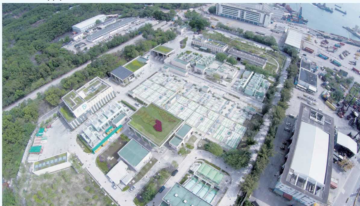
The Pillar Point Sewage Treatment Works
