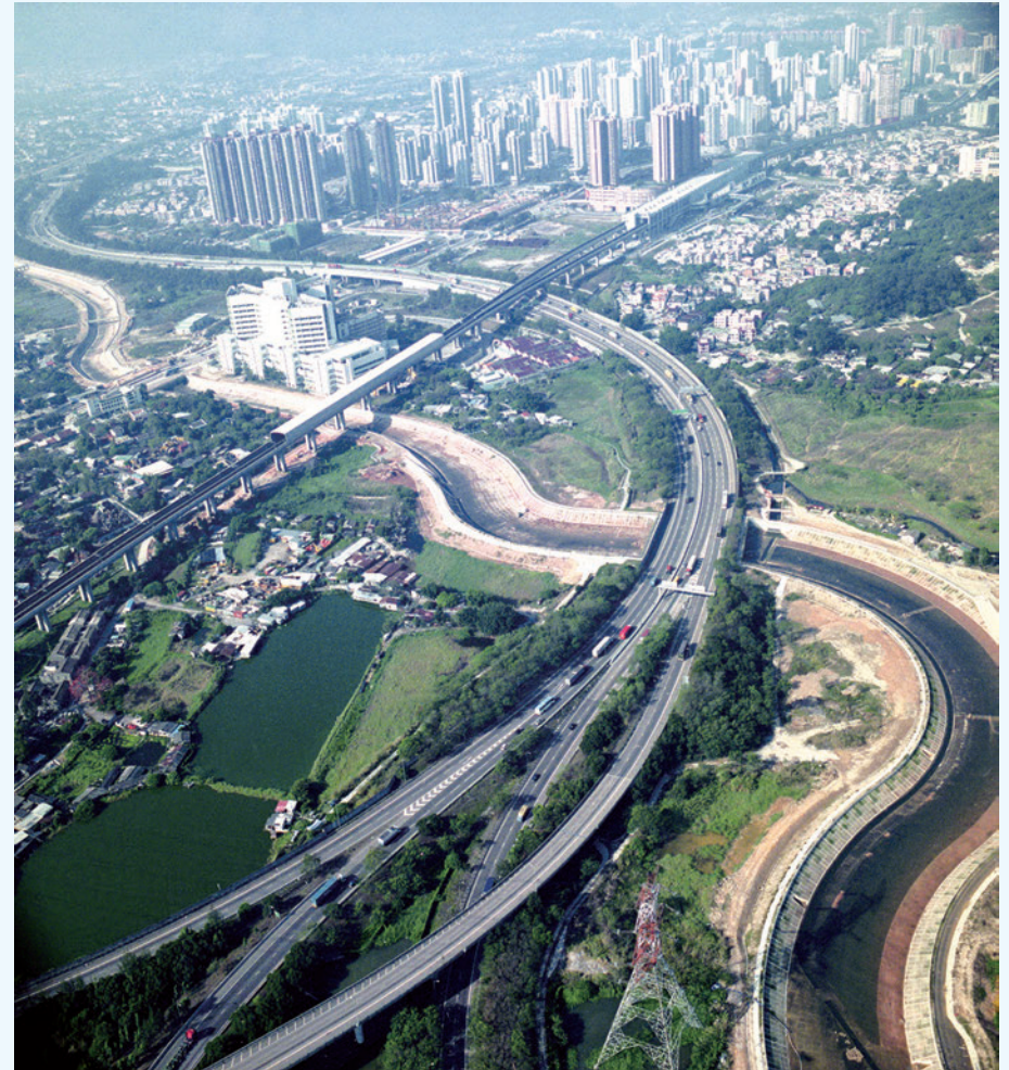
Construction of the Yuen Long Drainage Bypass in full swing in 2004
