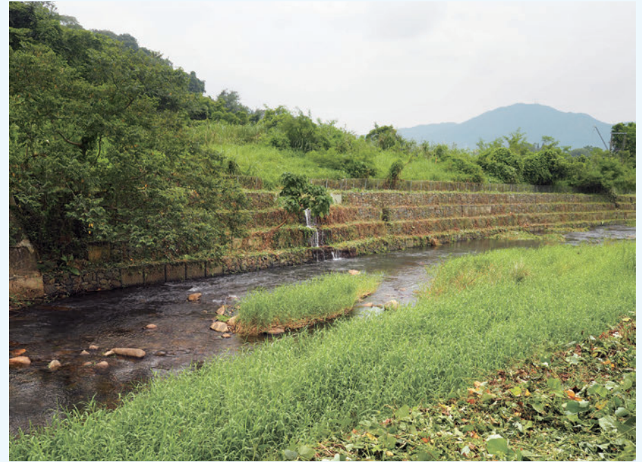
The Lam Tsuen River uses natural material for riverbed and gabion baskets for river bank
