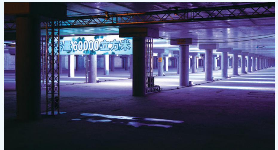
The Happy Valley Undergruond Stormwater Storage Scheme with a flood storage capacity of 60 000 cubic metres
