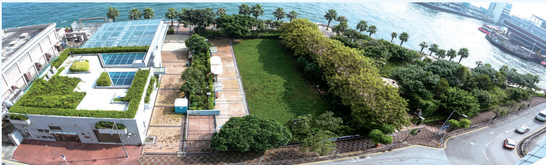
The pump house (left) under Sheung Wan Stormwater Storage Scheme and the landscaped open space above the underground flood storage tank (from middle to right)
