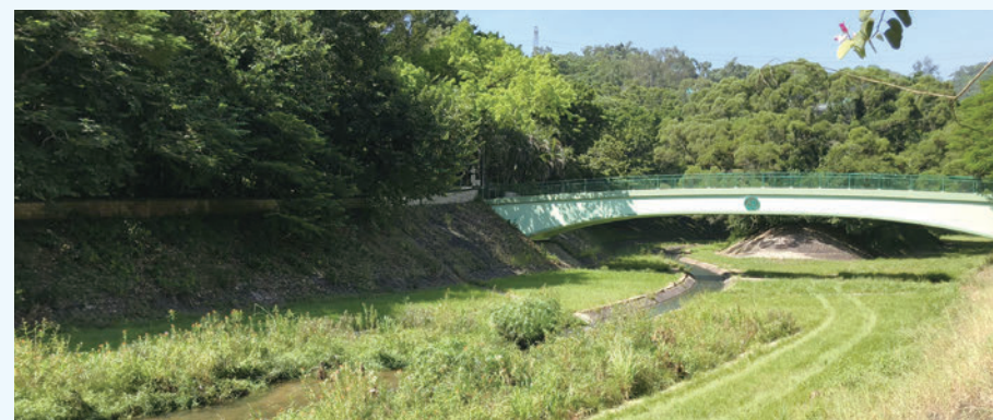
The riverbed and riparian zone of this section of Lower Lam Tsuen River has been given a new look after revitalisation using natural materials to replace the original concrete
