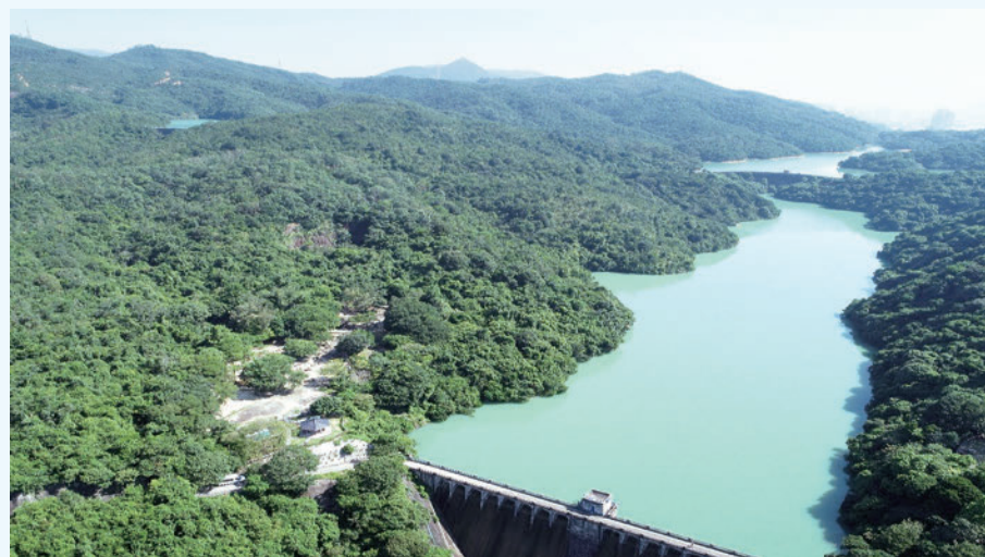
The proposed water intake will be overlooking at the Grade II historic structure of the Kowloon Byewash Reservoir Dam
