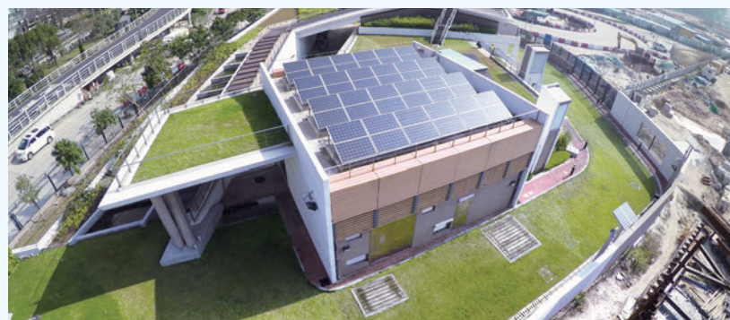
The Kowloon City Sewage Pumping Station No.1 bestowed the highest BEAM Plus Final Platinum rating for New Buildings
