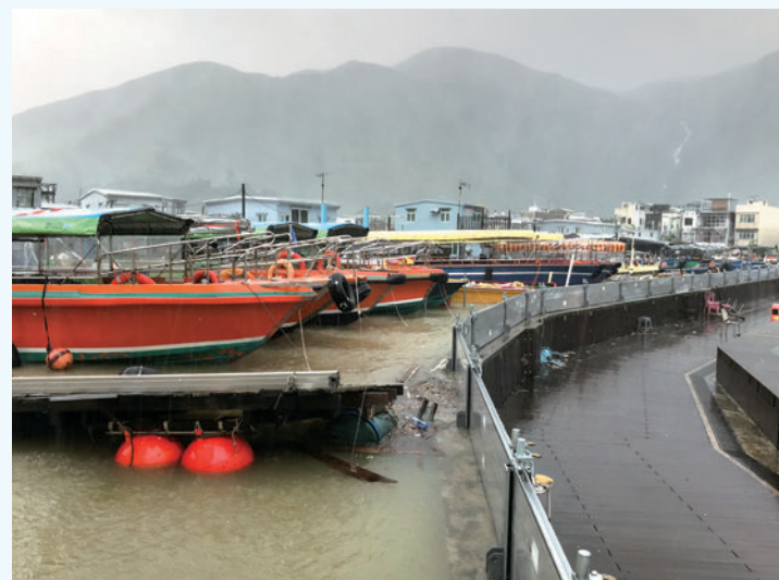
Demountable flood barriers have been installed in Tai O Creek along the river wall since 2014
