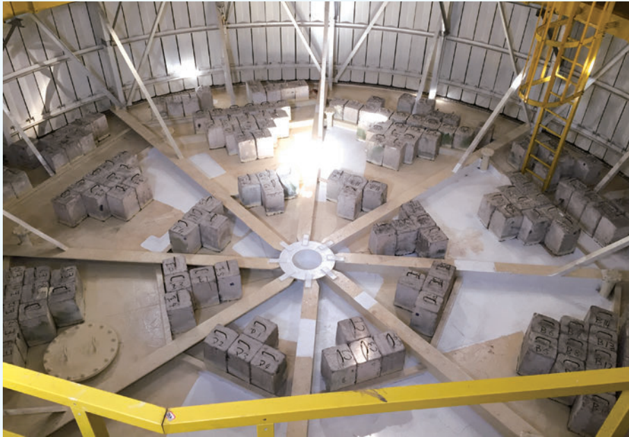
Interior of biogas storage tank
