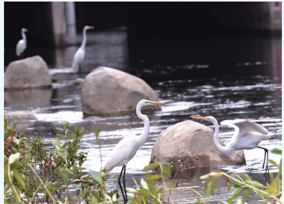
The use of natural materials for riverbed construction is a key element in the Revitalisation of Kai Tak River
