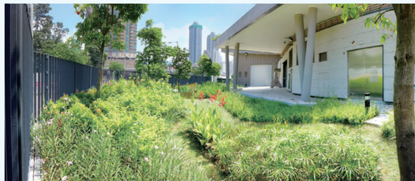
The rain garden inside the Kowloon City Sewage Pumping Station No.2 reduces runoff to the drainage system and uses the plants and soil to purify rainwater
