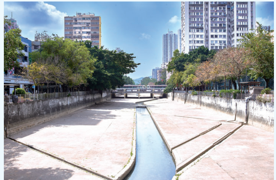
The heat island effect study has found that the surface temperature over concrete channel bed under sunlight could be as high as 62°C
