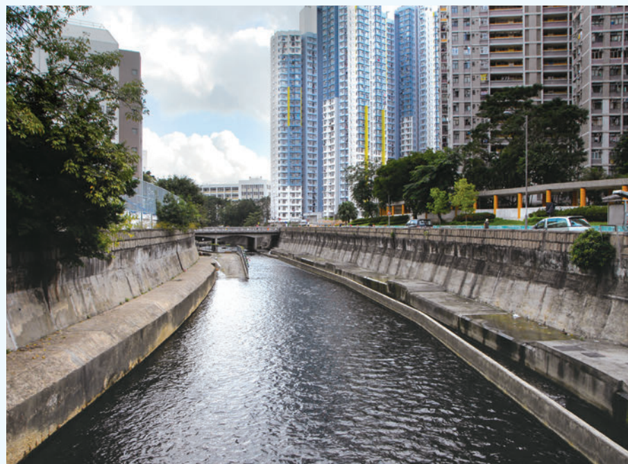
The Kai Tak River before river revitalisation
