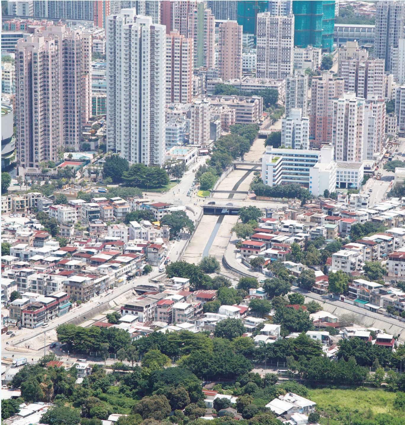
The Yuen Long Main Nullah built in the 1960s and 1970s were designed for fast flood relief. Aesthetic or ecological factors were secondary considerations.
