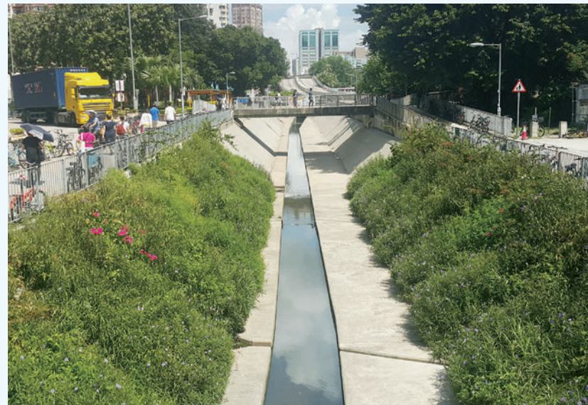
Pilot planting the urban on concrete embankments at the Yuen Long East Nullah provides urban greening and mitigates the urban heat island effect
