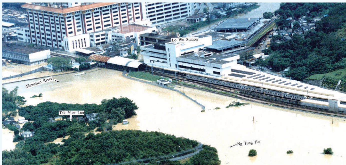
In the aftermath of Severe Tropical Storm Becky, which struck Hong Kong on 17 September 1993, Shenzhen River in the vicinity of Lo Wu and Ng Tung River were seriously flooded.
