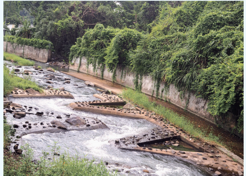
Fish ladders allow fish and other aquatic creatures to travel between the upstream and downstream of the river
