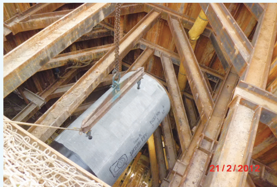
A jacking pipe is being lowered into the launching shaft
