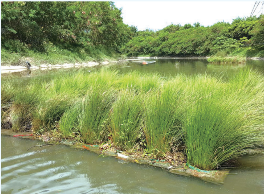
The planting raft at the Yuen Long Bypass Floodway on trial basis commenced in 2017, providing rest places for birds in deeper river channels
