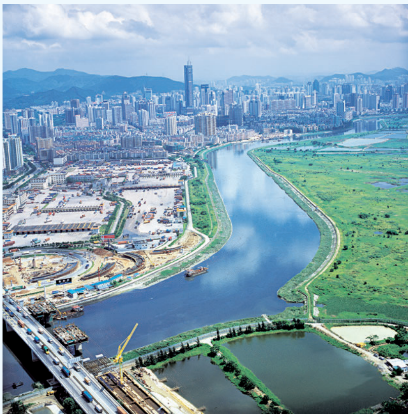
Completion of Stage 1 of Shenzhen River Regulation Project in April 1997 was followed by commencement of other cross-border infrastructure projects
