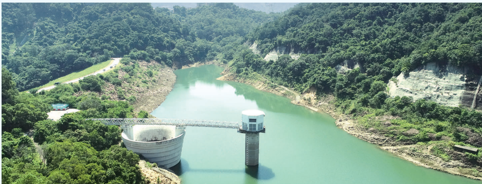
Outfall structure will be built at the Lower Shing Mun Reservoir at the end of the 2.8 kilometres long water tunnel
