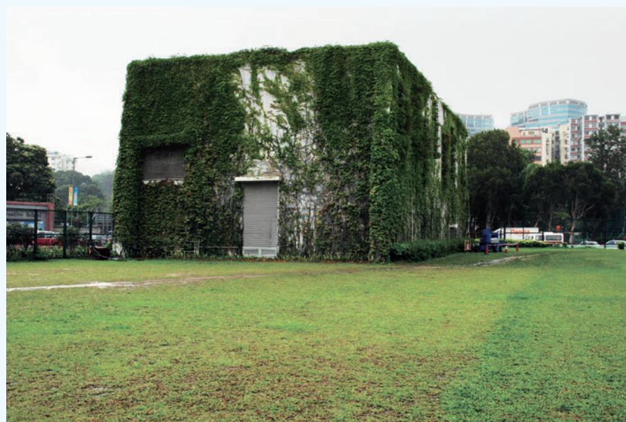
The first vertical greening undertaken by the DSD, completed in 2006 at the Tai Hang Tung Flood Storage Scheme.
