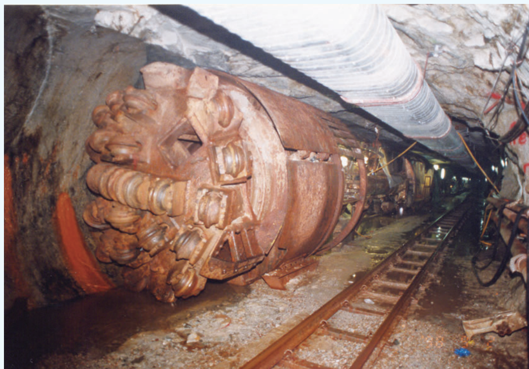
Tunnel boring machine (TBM) for HATS Stage 1 tunnel construction
