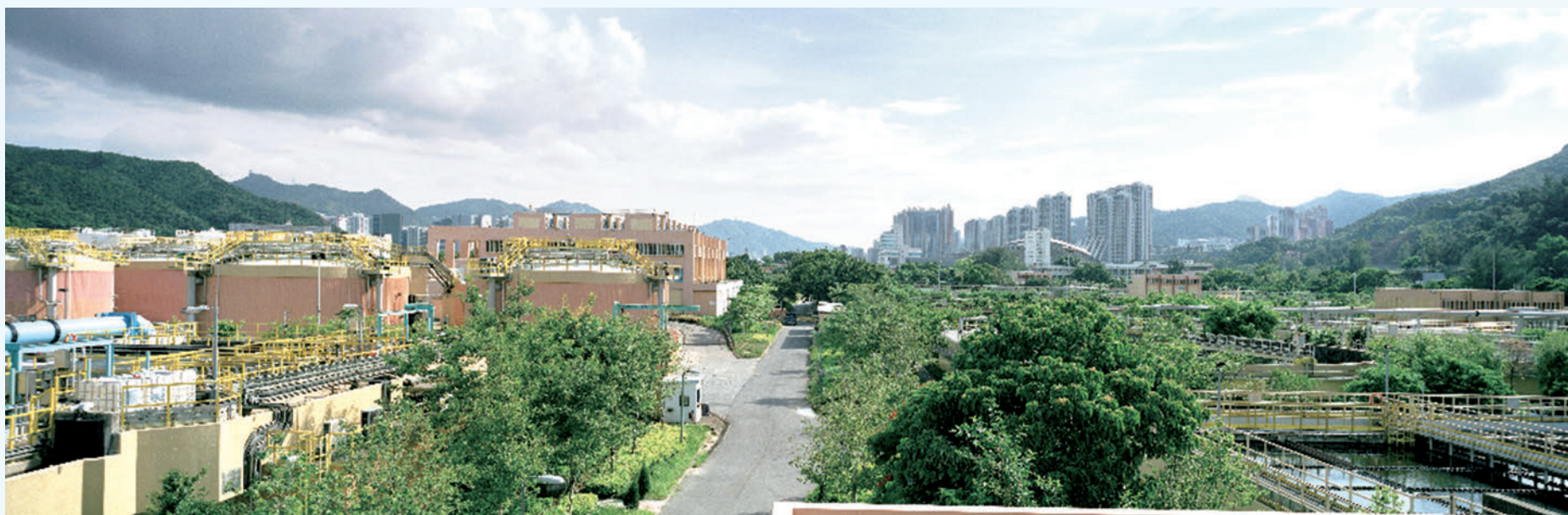
Sha Tin Sewage Treatment Works. The DSD has drawn up programmes for preventive inspections and maintenance, and contingency plans for possible emergency situations.
