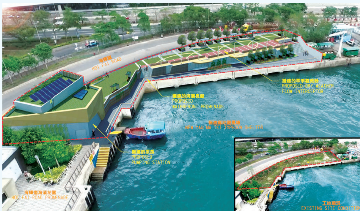
Photomontage of the dry weather flow interceptor at the Cherry Street Box Culvert and its promenade
