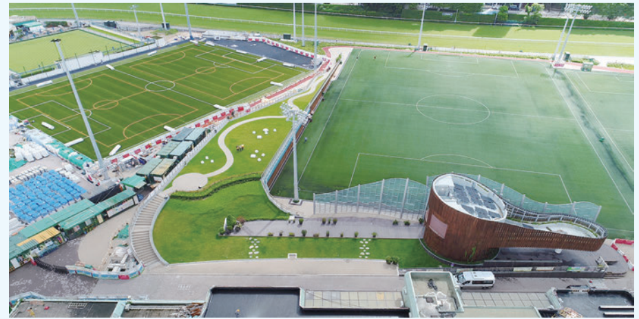
The landscaped mound on the rooftop of the pump house (left) and the fan room (bottom right) blend in harmony with the surrounding environment and provide leisurely space for the public
