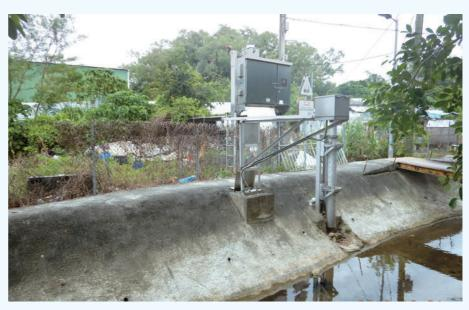
The DSD has installed flood alarm systems to alert the local villagers at flood-prone areas before drainage improvement works are completed
