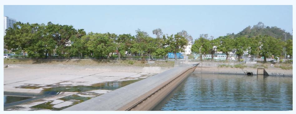
Inflatable dam in Yuen Long Main Nullah near Tung Tau Wai was constructed in 1992 to prevent polluted tidal water from backflowing into the Yuen Long town centre
