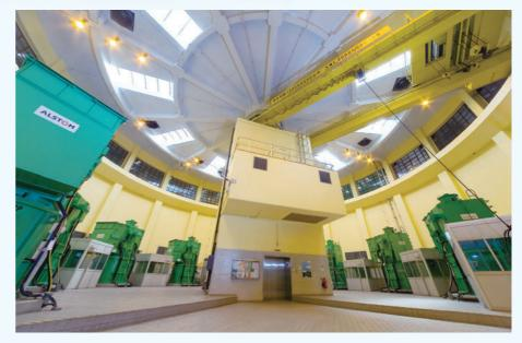
Eight sewage pump motors installed in the Main Pumping Station No. 1 at the Stonecutters Island Sewage Treatment Works under the Harbour Area Treatment Scheme
