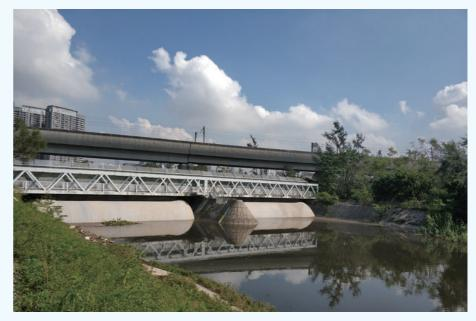
Inflatable dam at San Tin Eastern Main Drainage Channel near its confluence with Shenzhen River, the highest inflatable dam in Hong Kong with a 5 metres full height.
