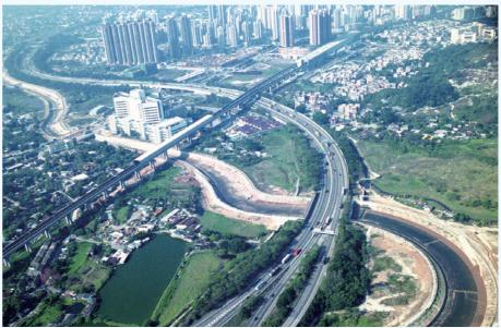
Yuen Long Bypass Floodway diverted part of the runoff from Yuen Long town centre to Kam Tin River east of Yuen Long to reduce the risk of flooding in the Yuen Long Town
