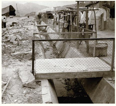
Open channels at Kwai Chung Licensed Area (left) and stormwater drains at Kowloon Tsai squatter area (right) during late 1960s. At that time, environment issues of any drainage services were seldomly accounted for.
