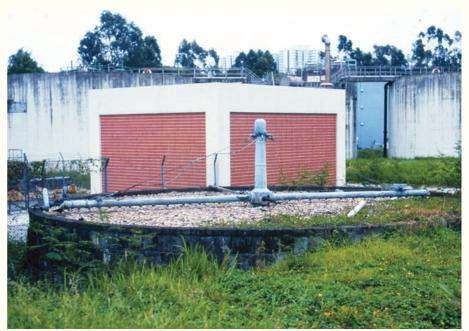
Trickling Filter of the Shek Wu Hui Pilot Sewage Treatment Plant
