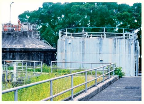
Anaerobic Sludge Digester of the Shek Wu Hui Pilot Secondary Sewage Treatment Plant
