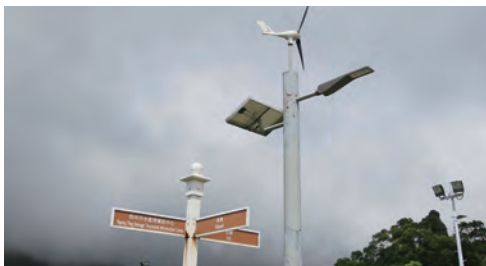
Solar-wind power lamp poles at Ngong Ping Sewage Treatment Works for lighting
