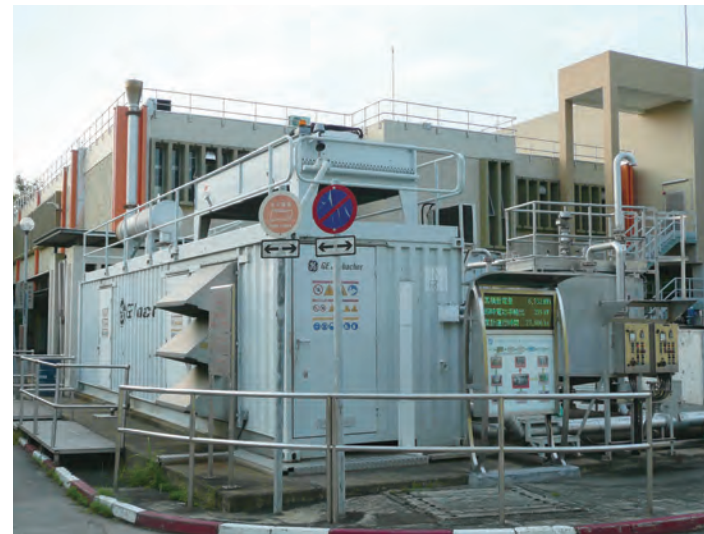
CHP generator at Shek Wu Hui Sewage Treatment Works
