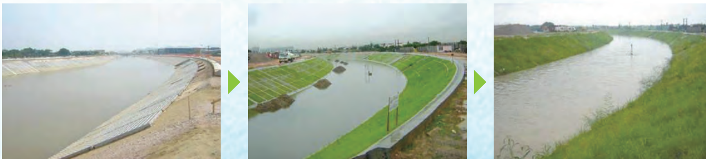
Procedures for laying grasscrete along Ngau Tam Mei Main Drainage Channel
