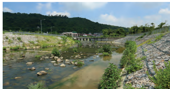
Gabions provided along the embankments of Lam Tsuen River
