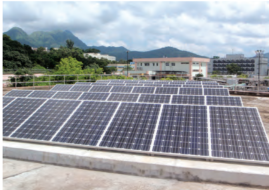
The solar photovoltaic system at the roof top of Yuen Long Sewage Treatment Works provides partial electricity supply for the plant by grid-connection
