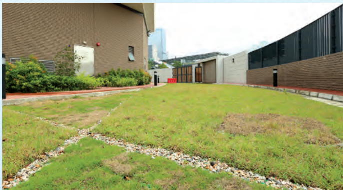
Grass paver was used to pave the emergency vehicular access of Kowloon City Sewage Pumping Station No. 1
