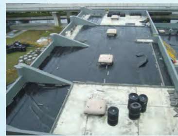
Install root barrier
