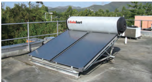
The solar water heater at Shek Wu Hui Sewage Treatment Works supplies hot water for daily use
