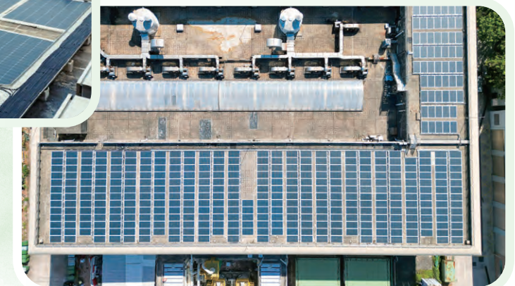
◀ 設於西北九龍基本污水處理廠的柔韌單晶硅太陽能發電系統 Flexible Monocrystalline Photovoltaic System at North West Kowloon Preliminary Treatment Works
