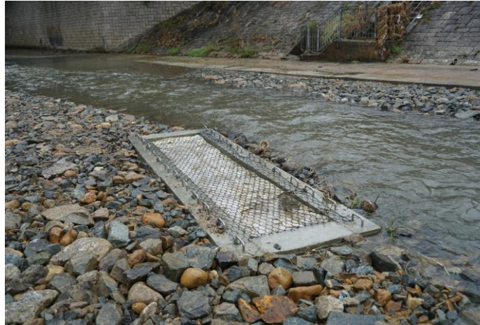
Current Deflector Installation
