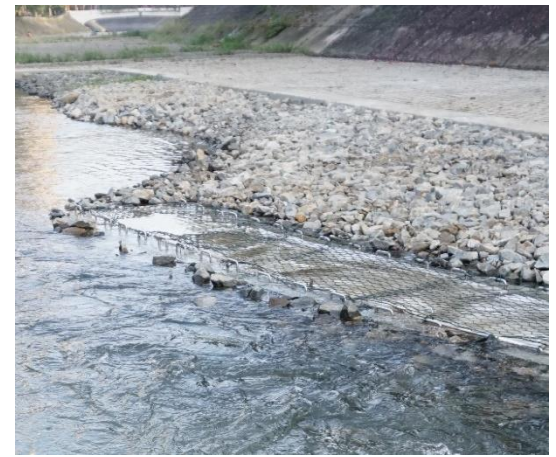
Current Deflector Installation
