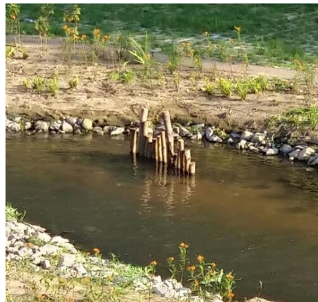
Wooden Poles Installation
