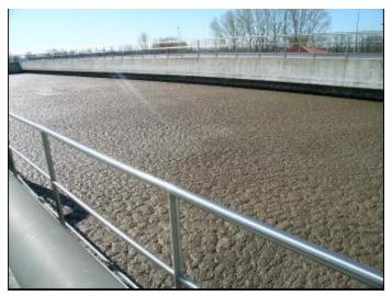
Foam and bulking in the activated sludge process at WWTP Lariana, Italy [Fabiyi et al. 2007] **<u>Client:</u>** WWTP Lariana, Bulgograsso, Italy
