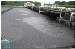
Foam and bulking in the activated sludge process with ozonation in operation [Fabiyi et al. 2007]
