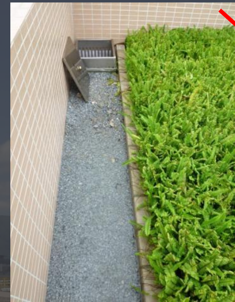
Drainage Inspection Chamber
