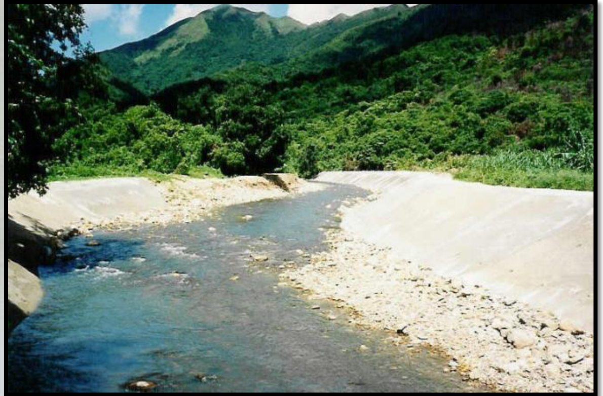
After river training works
