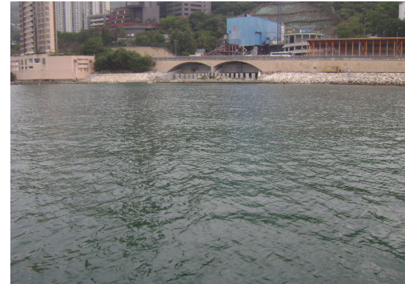
Photographic record for exceedance of Dissolved Oxygen (marine bottom) recorded at O-1(FT) on 30-Mar-12
