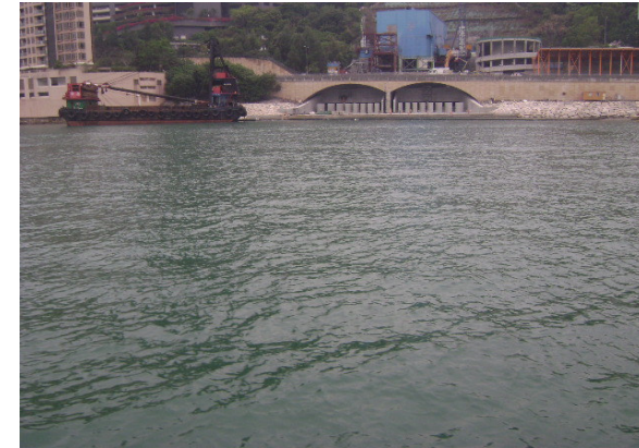
Photographic record for exceedance of Dissolved Oxygen (marine bottom) recorded at O-1(FT) on 23-Mar-12
