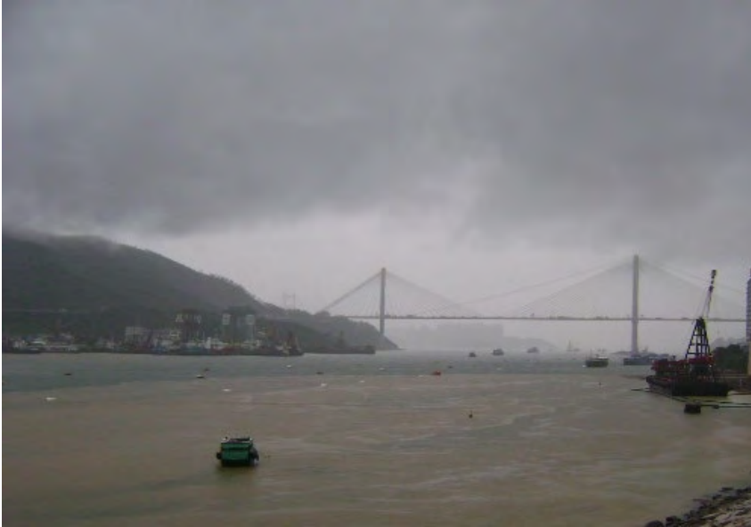
Site photo (Photo taken at location near Greenview Terrace)
