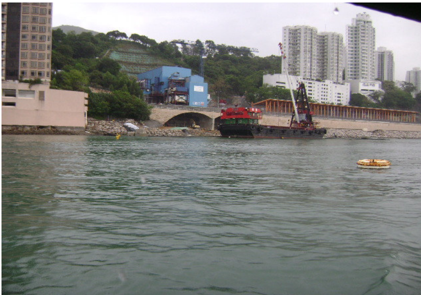
Site photo (Photo taken at location near O-1-C(ET))
