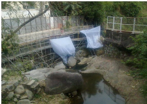
Construction activities at I-2-C.
