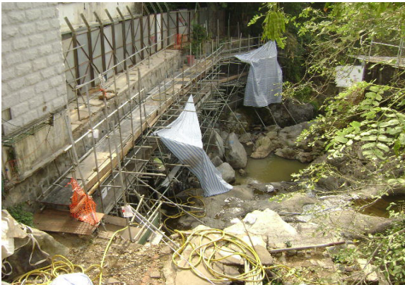
Construction activities at I-2-C.
