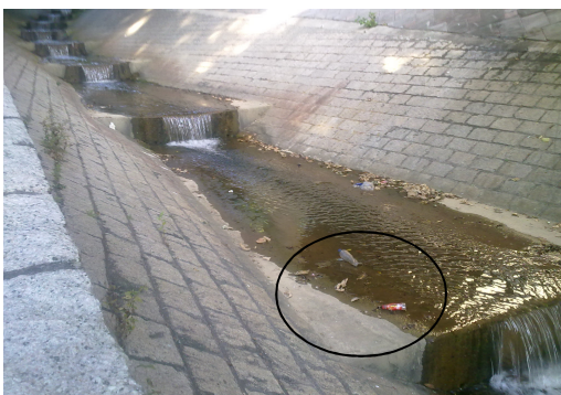
Rubbish was observed at I-1-C
