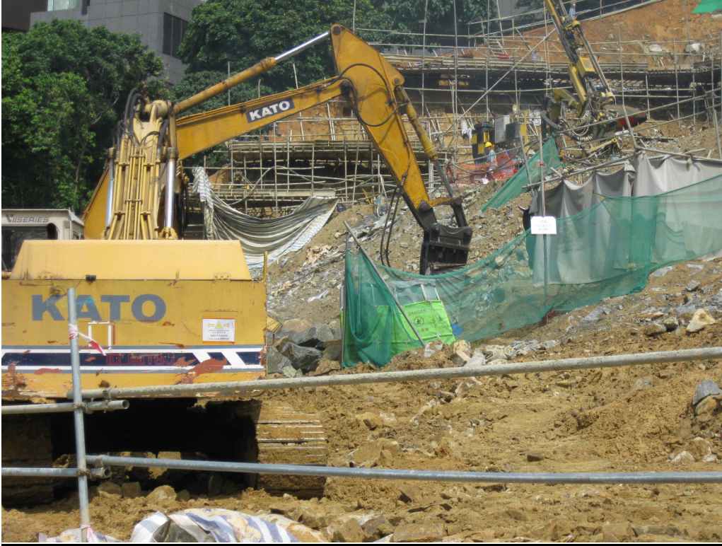
3. Noise insulation material for rock breaking.
