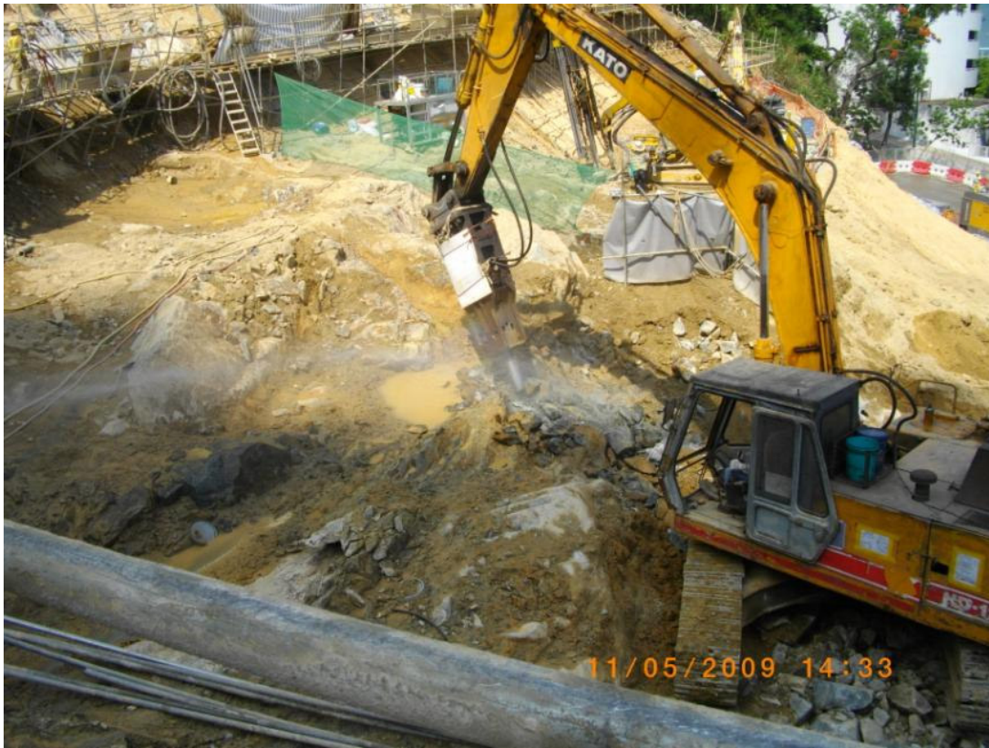
3. Water spraying during rock breaking.
