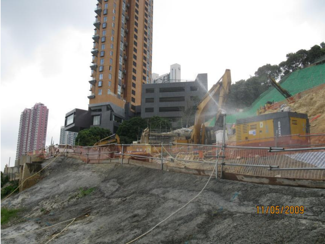
1. Water spraying for the exposed area.
