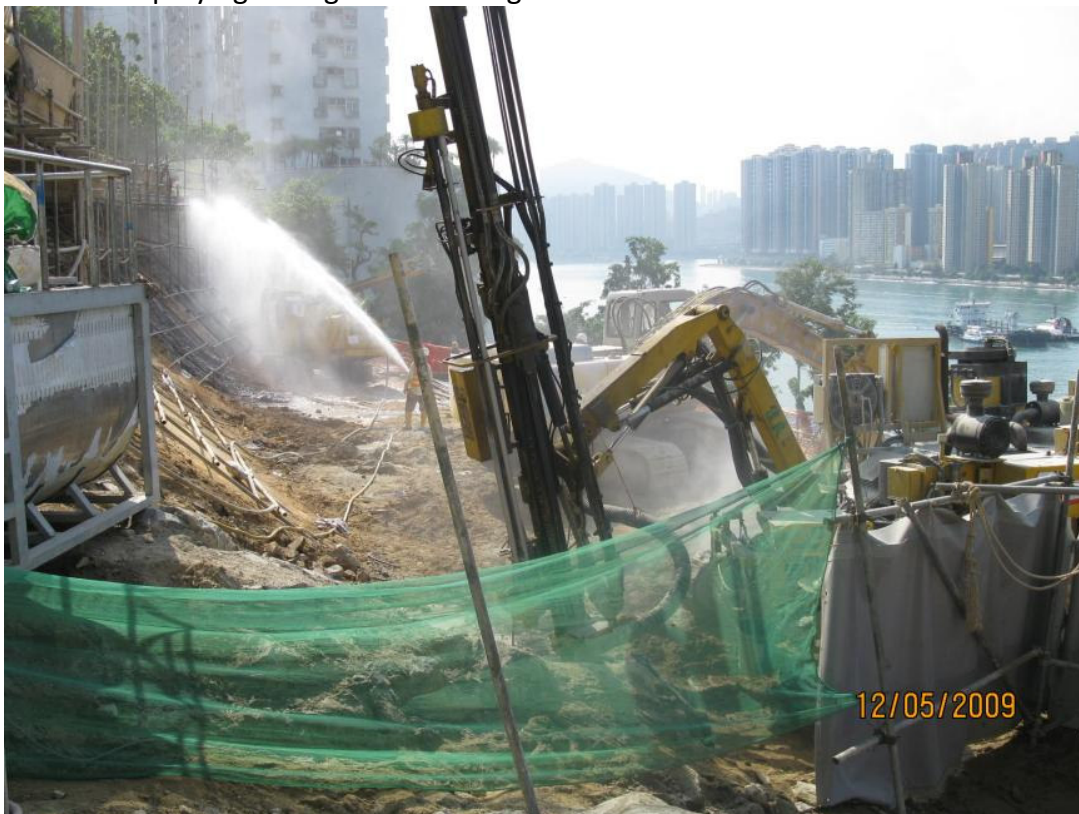
4. Water Spraying for soil nail work.
