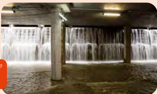
Demonstration of the movable weirs' operation 可調式溢流堰的操作示範
