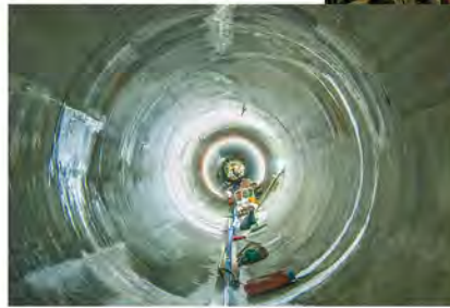
昂船洲隧道 Tunnel at Stonecutters Island
