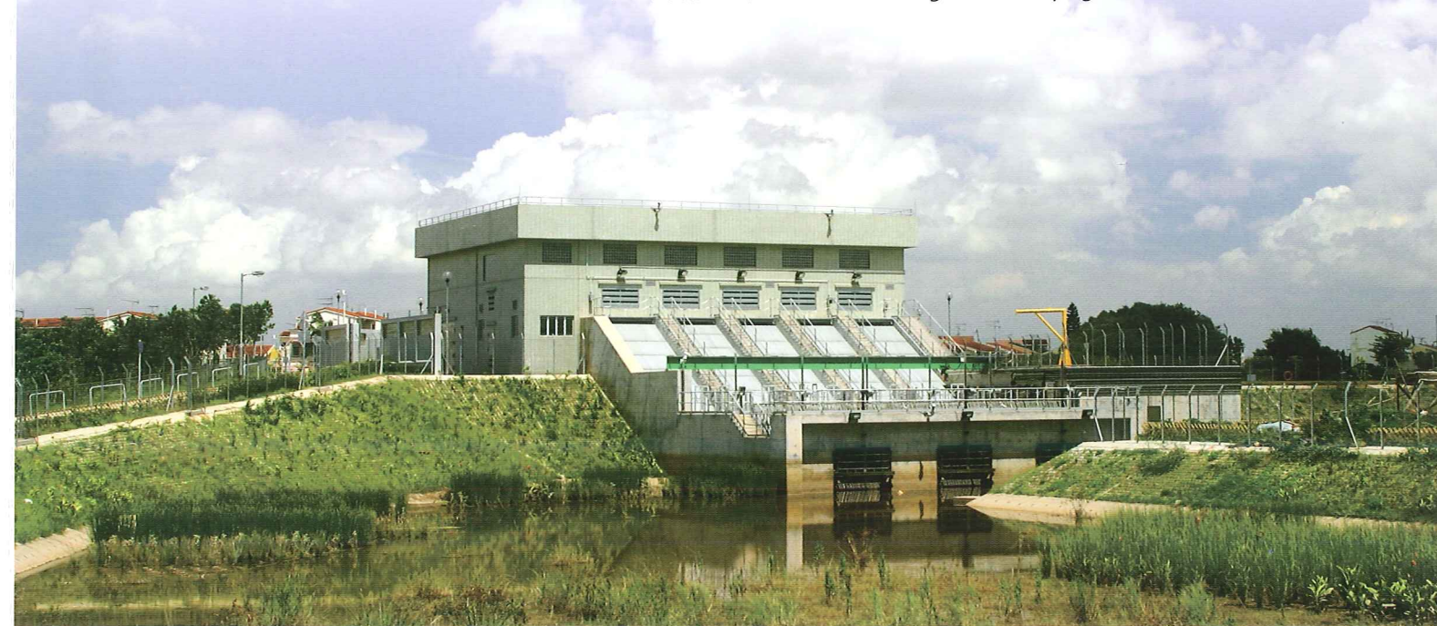
位於竹園村的鄉村防洪抽水計劃 Village Flood Pumping Scheme at Chuk Yuen Tsuen
