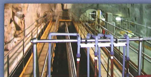
消毒槽 Disinfection Channel
