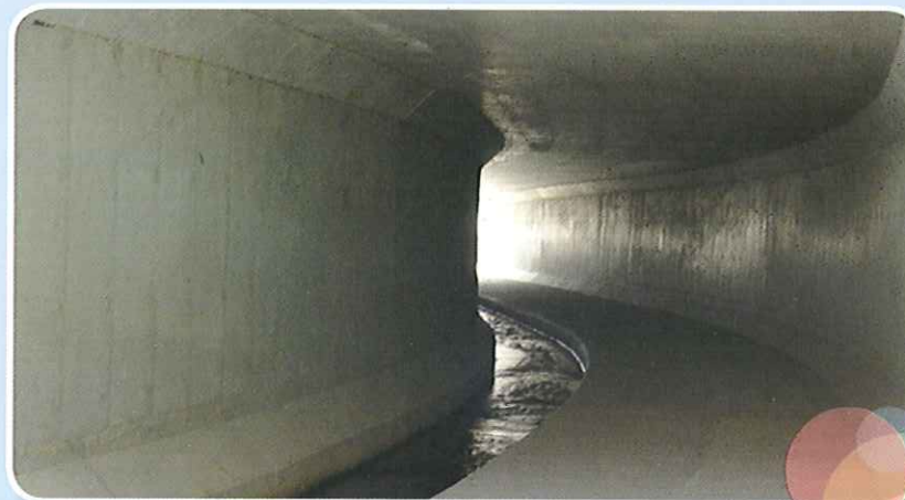
排洪暗渠 Drainage Culvert
