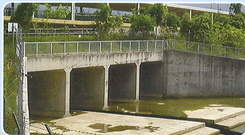
排水道出口 Outlet of a Drainage Culvert
