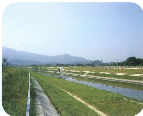
新田東排水道 San Tin Eastern Main Drainage Channel
