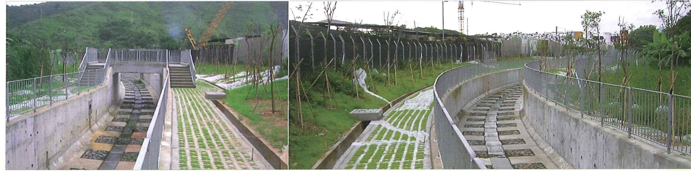
打鼓嶺水流坑的矩形雨水明渠 Rectangular drainage channel at Shui Lau Hang, Ta Kwu Ling
