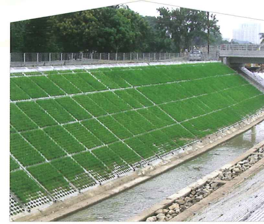
新河道面的草磚 Grasscrete panels on the new river channel
