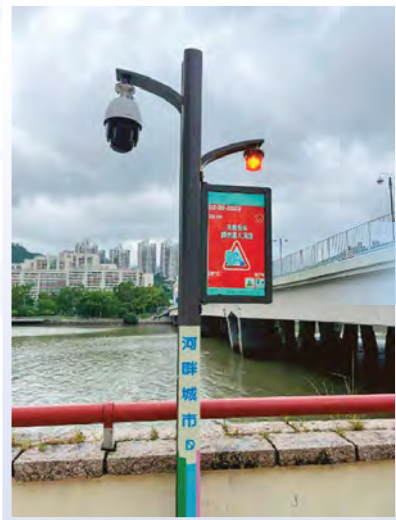
主要行人通道旁邊的智能桿 Smart pole next to the main pedestrian passage along the river
