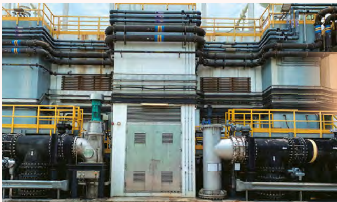
昂船洲污水處理廠的水力渦輪發電系統 Hydro-turbine generating system at Stonecutters Island Sewage Treatment Works
