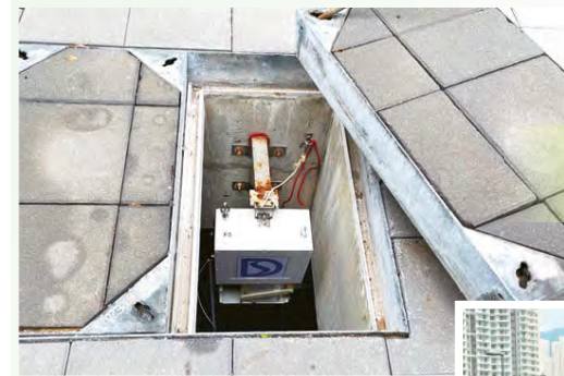
沙井內自動採樣裝置的安裝 The deployment of the sampling robot in the manhole
