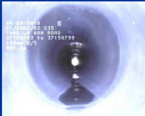
CIPP (Cured-in-Place Pipe)
