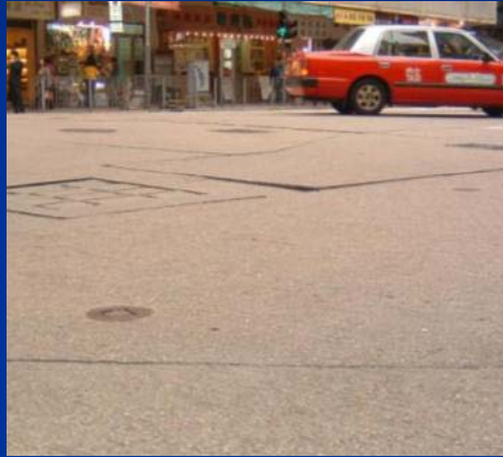
Crack & Stepping
